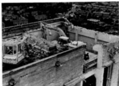
Concrete breakers and hydraulic cutters at work
