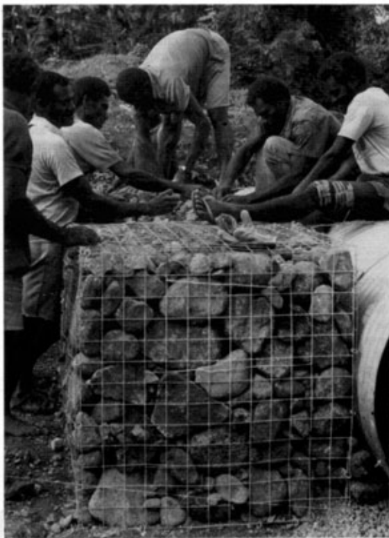
Photo 1. Local labour filling gabion baskets by hand
