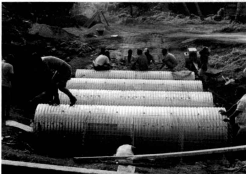
Photo 2. Armco culverts for an Irish bridge
