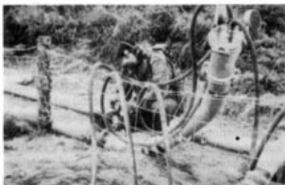
Sgt Joyce, 516 STRE(BP) fitter, checking fuel pipeline prior to compressed air pigging
