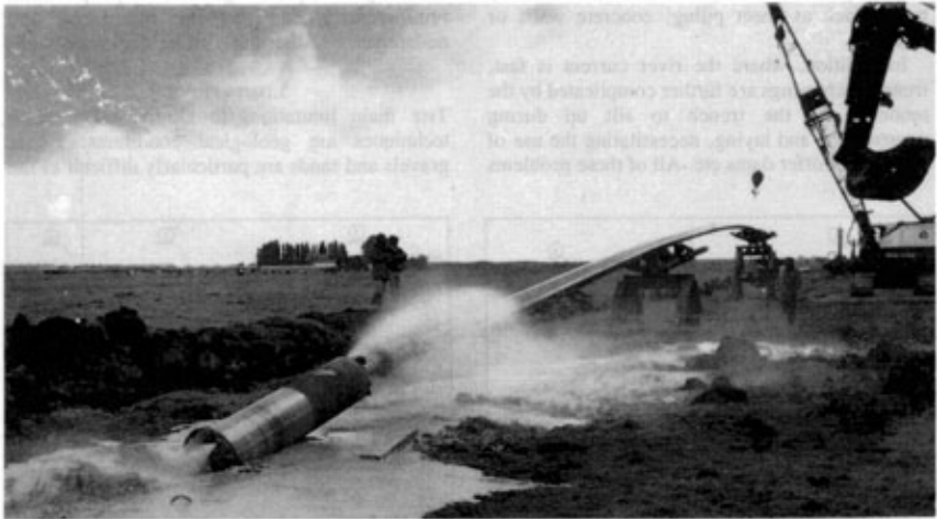
Figure 9. Jet reamer in action
