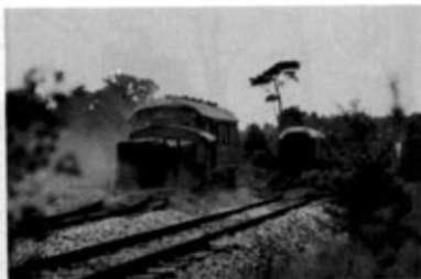
The impetus of the locomotive lifts the track in front of the crater
