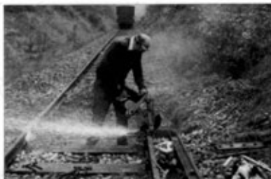
A member of the PWT cutting out damaged rail
