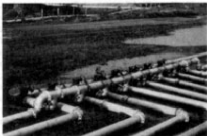
Aviation fuel tank manifold in shore storage area
