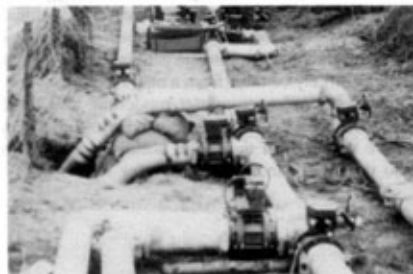
The shore storage splitter manifold. This handled fuel from the raft-mounted pump station and also fuel storage to the airhead.
