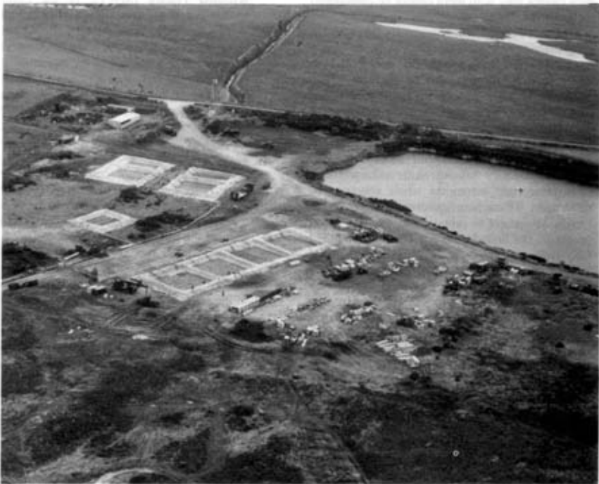
Photo 2. EX PURPLE WARRIOR—Scotland Nov 87. The construction of the beach storage bunds, tanks and pipework prior to fuel being pumped ashore over the beach via a pump raft fed by towed flexible barges filled from an RFA tanker offshore. The fuel system replenished Phantoms, Harriers, helicopters and vehicles during the exercise.
