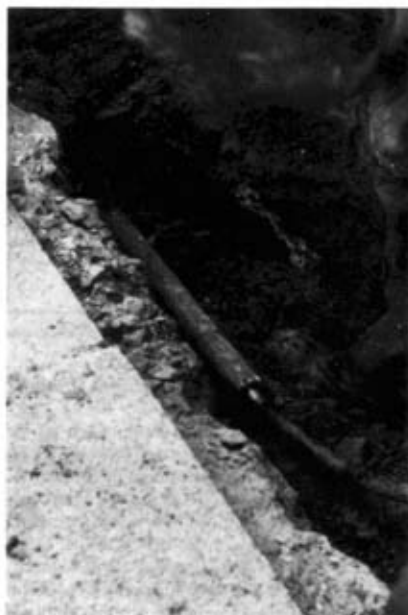
Photo 3. 45mm mole in launch pit at start of bore
