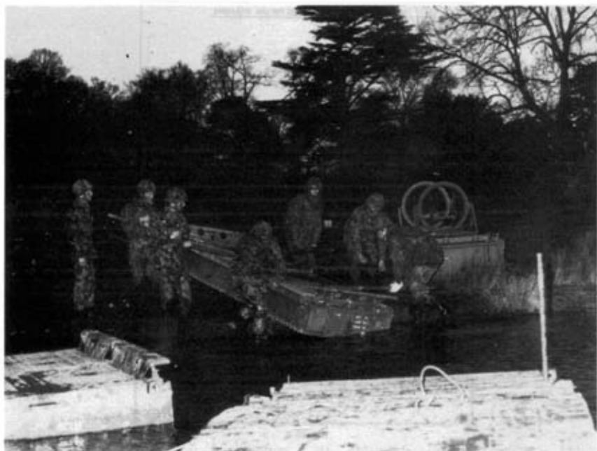
Photo 1. Men from 20 Fd Sqn building an APB raft prior to a night ferry operation, during a 36 Engr Regt exercise on Stanford Training Area.
