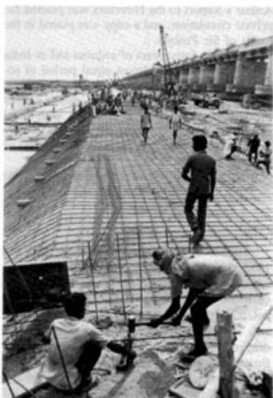
Photo 4. Work in progress on repairing the damaged section of the original anicut (courtesy Newsline ).
