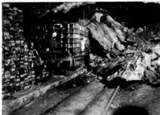
Photo 2. View of the collapsed state of the tunnel system of the Old Store believed to have been taken after the accident.
