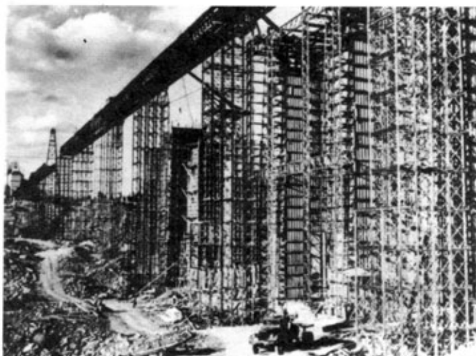
Photo 8. Extensive use of Bailey for temporary works on a hydroelectric project in Canada in the late 1940s.
