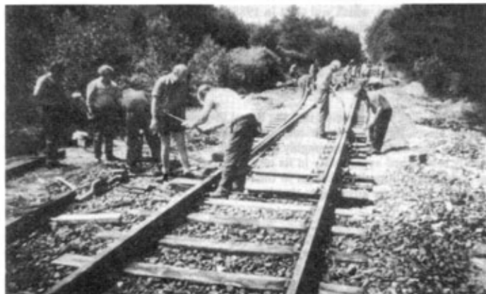
Photo 7. 507 STRE constructing a length of permanent way at Bracht during their annual camp.
