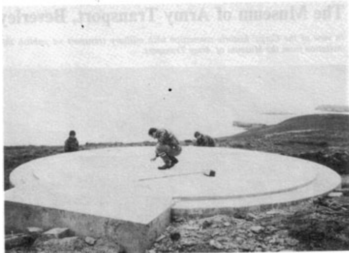
Photo 2. Finishing off the concrete pad.
