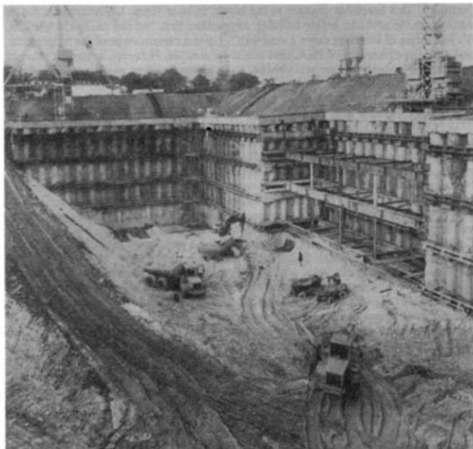
Photo 2: Diaphragm wall-building—the early stage of WHQ construction.
