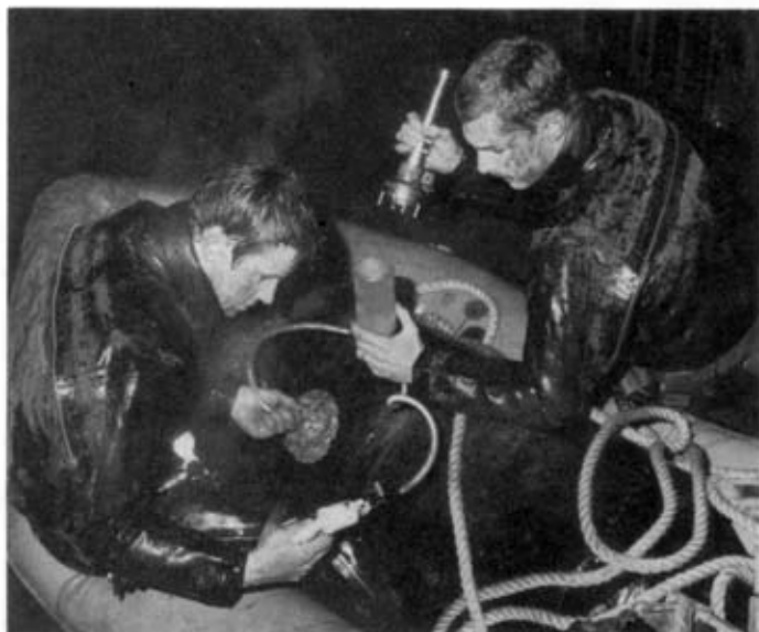
Photo 2. Major Hall immunises the fuze whilst Sapper Wright holds the torch.
