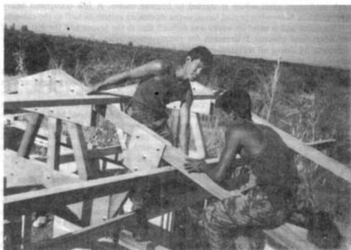
Photo 1. Roof purlin being fixed.
