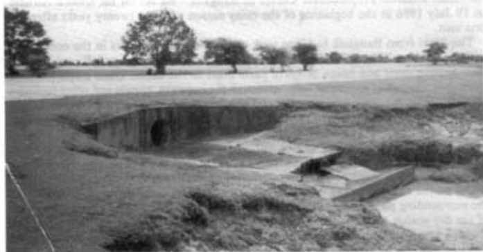
Photo 2. Culvert under taxiway.
