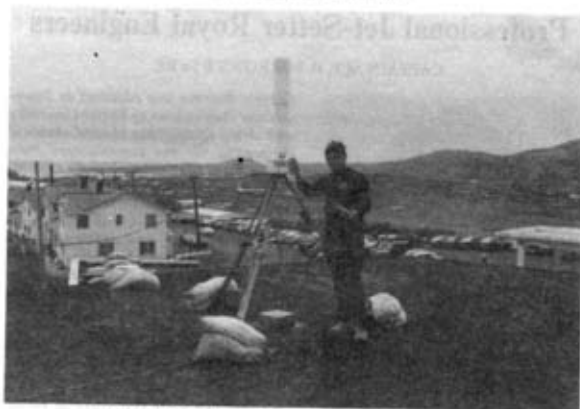
Photo 1. SSgt Al Barnes RE guying the antenna on the Azores.
