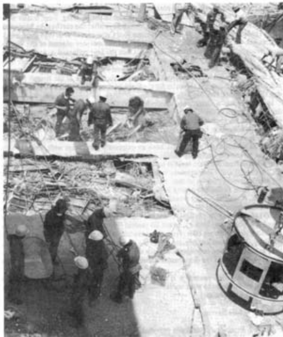
Photo 1. Removal of the roof by cutting out slabs followed by beams.
