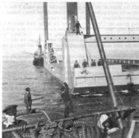
Photo 3. Preparing to locate a pierhead in position.
