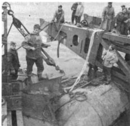
Photo 4. Coupling up the bridge in bad weather. Note erection tank. Sergeant Blake in foreground.
