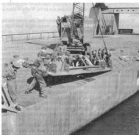
Photo 6. On the pierhead. Preparing seating for the bridge end.
