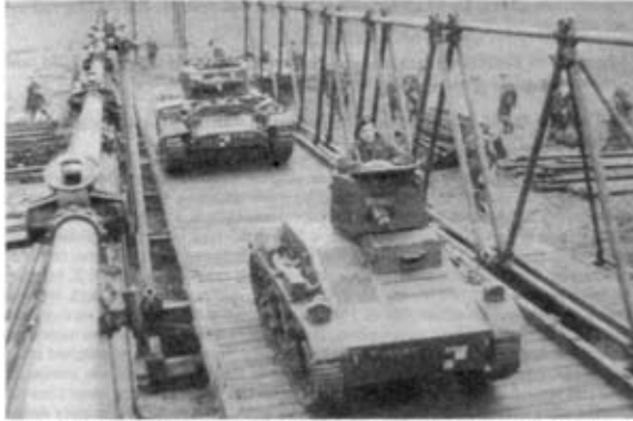
Photo 2. Light tanks crossing a Mark III Inglis bridge; note the knee bracing and the use of the extra truss members at mid-span.
