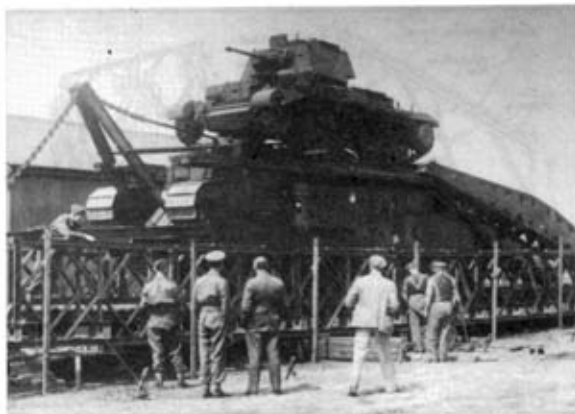
Photo 3. A Double/Single bridge under test load in early 1941. Donald Bailey is in the foreground, in his familiar sports jacket and cloth cap.
