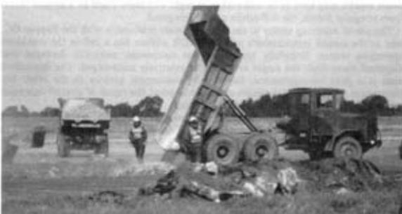
Photo 4. Placing the fill
