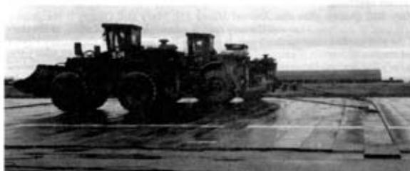
Photo 3 MWT's carrying out an AM2 mat straightening operation on RAF Stanley. Bowing is clearly visible in the row in front of the strop anchor points.
