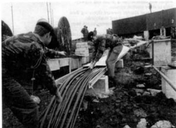
Photo 6 Laying electrical cables in ladder racking during the further development of the Project *ZEUS* site
