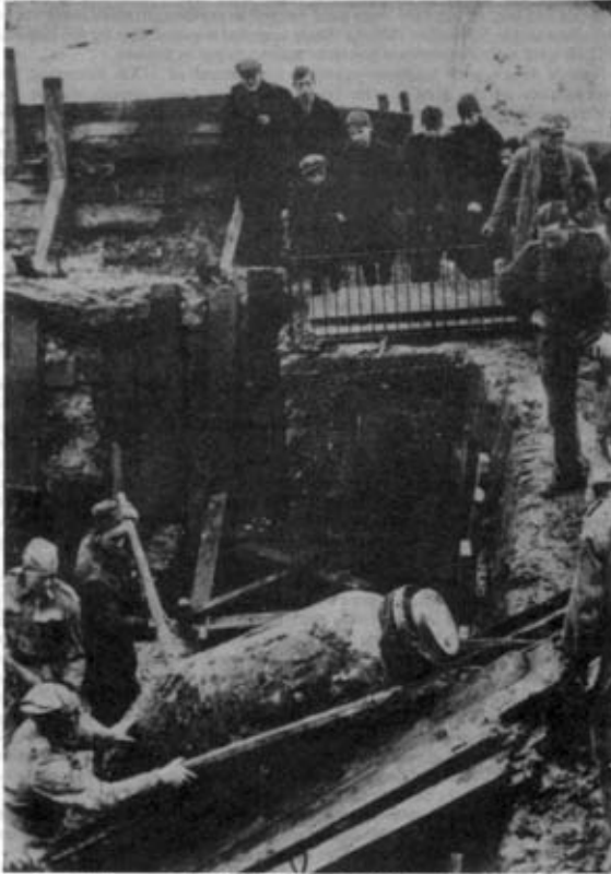
Photo 1. Typical scene around 1940/1941 "Hermann" 1000Kg bomb being dragged from a shaft after the fuse had been immunised. (London Church Yard)
