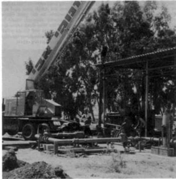
Photo 3. El Farajh Pump Station—withdrawing 250m of pipe
