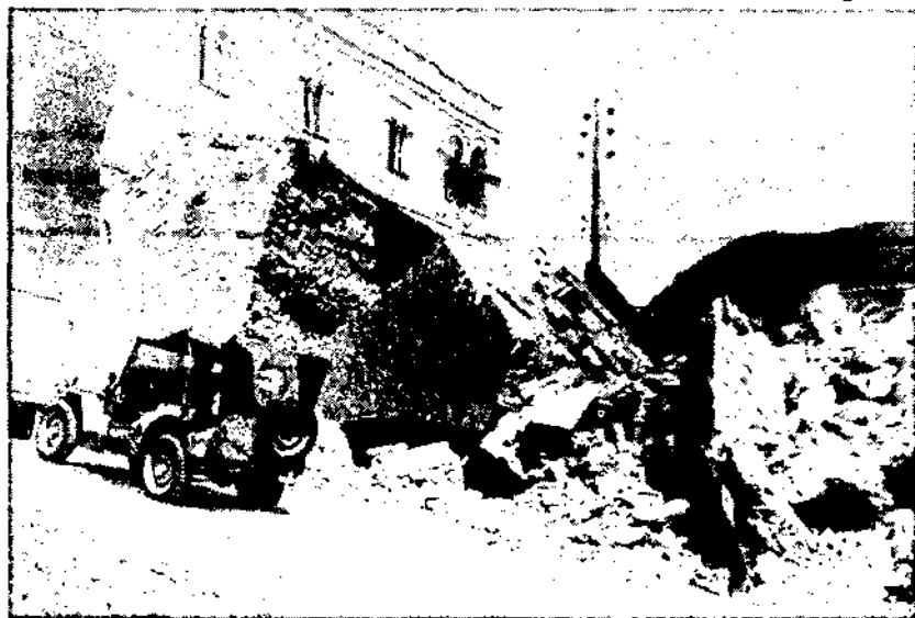
Photo 2. The temporary track to bypass the debris of the demolition
