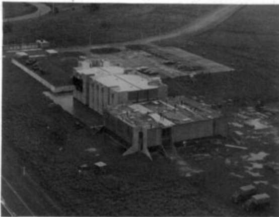
Photo 6. Approx Day 70. Commencing roof sarking. Continue erection East wall which incorporates long run steel for future extension if required
