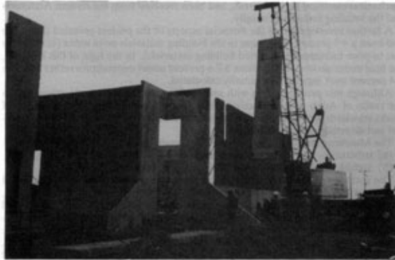
Photo 2. Day 40. Last wall panel is swung into position
