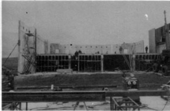
Photo 5. Day 50. Looking West. Showing boxing to concrete beam and edge of Dycore flooring
