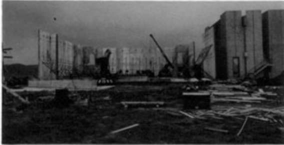
Photo 3, Day 43. Panel walls complete. Commencing erection mezzanine floor posts and beams
