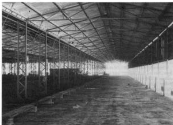
Photo 8. Our first light steel for much needed shedding. Steel rolled in the repaired and forces operated steel mill in Bari (25ft span \times 14ft high)
