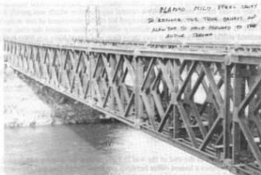
Photo 9. Flambo mild steel Bailey designed by John Lander. First bridge erected across Dead Horse Gap, Class 30, 100ft span
