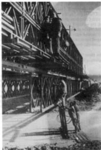
Photo 2. The first Triple Bailey ever built
