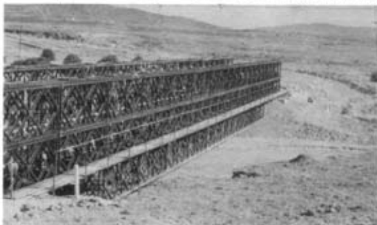
Photo 1. The first Triple Bailey ever built under construction
