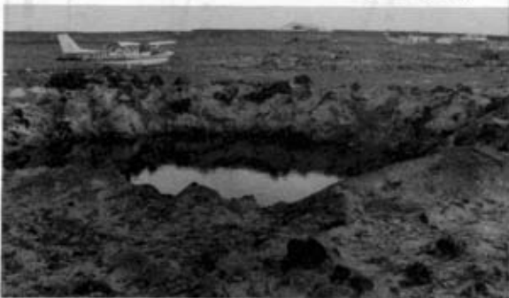
Photo 1. Crater on edge of runway caused by 1000lb bomb from Vulcan. Also in the photograph is a damaged Islander aircraft, aircraft hangar and terminal building
