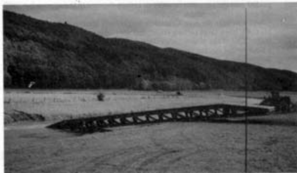
Photo 3. Delaunch of Medium Girder Bridge
