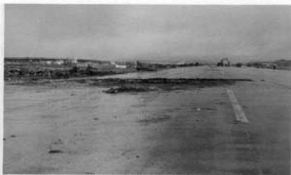
Photo 8. The Vulcan crater with most of the debris cleared. To the right of the photograph, repairs to the northern half are being carried out by 1 Troop 59 Commando Squadron
