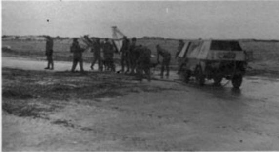
Photo 4. Sappers preparing Vulcan crater for repair by cutting back heaved area
