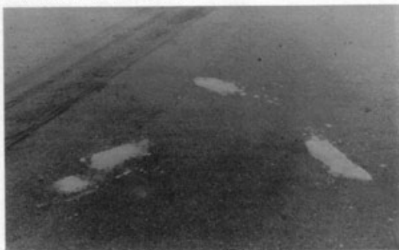
Photo 7. Scab being repaired with Bostik 276
