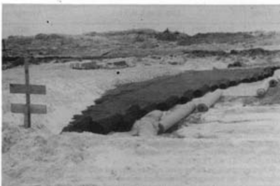
Photo 11. The use of geotextiles on the runway extension
