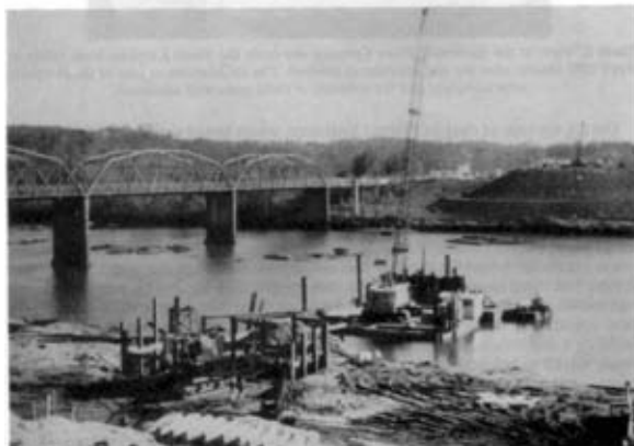
Photo 1. View of the Savannah River Crossing site from the Georgia bank taken early in November 1981, showing construction of the first two cofferdams in progress. The "Old" bridge, dating from 1926, is on the left, 200 feet upstream of the new alignment
