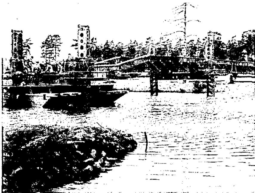
Photo 5. Piers in position ready to support bridge once boomed
