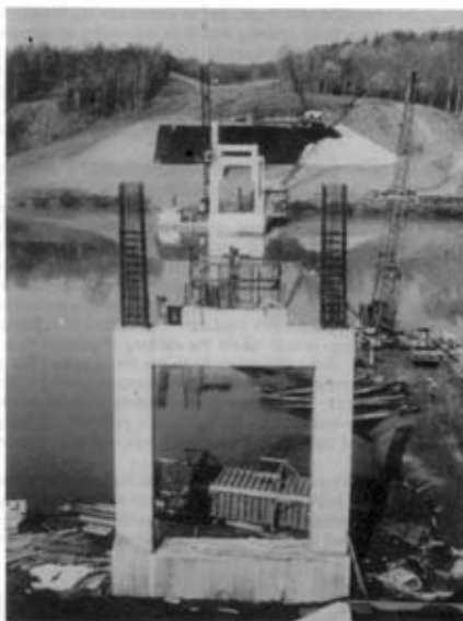
Photo 2. View of the Savannah River Crossing site from the South Carolina bank taken in April 1982 shortly after my site attachment finished. The foundations of four of the five piers were complete and the columns of three piers well advanced
