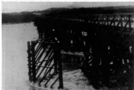
Photo 4. Early stage of the Imjin in spate. In spite of the "shear-waters" we lost a pier and two spans of this bridge a few days later
