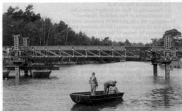
Photo 1. View of undecked bridge supported on two piers
