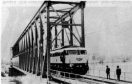
Photo 8. 120m span SKB erected as an emergency bridge over the R Toce in Northern Italy 1978. Acier-Stahl-Steel
