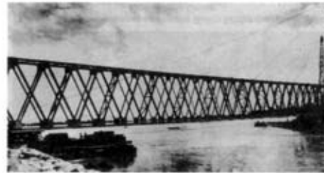
Photo 5. Single span 76m Type "C" Callender-Hamilton Bridge under construction over the R Manas, Assam in 1942. Balfour Beatty Power Construction
