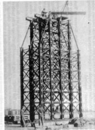
Photo 2. Standard trestling being erected.
