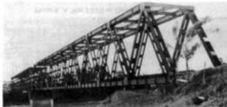
Photo 10. Two 82m Acrow Heavy Bridge spans. Acrow Group
