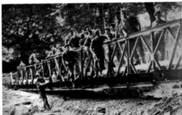
Photo 1. The main road bridge at Simonsbath after completion of Class 9 and during the operation of strengthening the bridge to take Class 30 road traffic (1952 West Country Floods)
