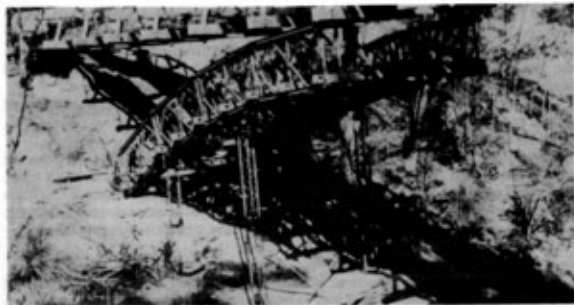
Photo 9. The main props have now been positioned and the construction continues by cantilevering out the bays. Note the old bridge is about to foul the arch
