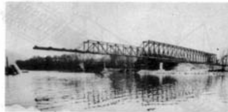
Photo 7. Launching a 120m span SKB. Acier-Stahl-Steel
