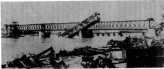
Photo 1. SKR-6 railbridge of three 91m continuous spans over the Rhine at Mannheim (1946). Acier-Stahl-Steel
