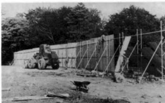
Photo 4. Part of the Cover From View (CFV) Fence nearing completion. Note the "Christmas Tree" lattice braced fence supports.
