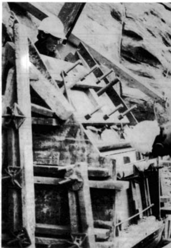
Photo 5. Final adjustments to formwork for arch thrust block being made
