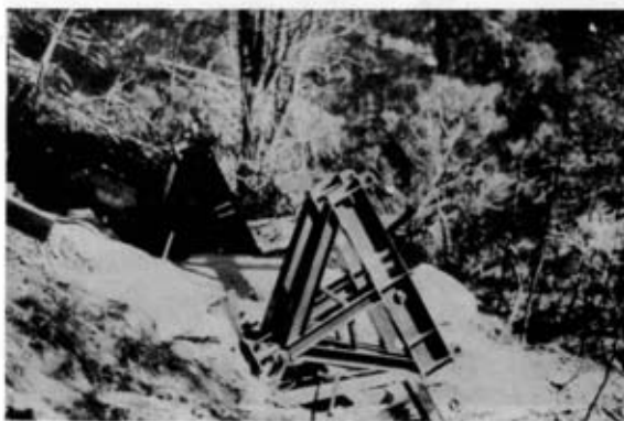
Photo 8. First angle panels in position and fixed to the base plate
