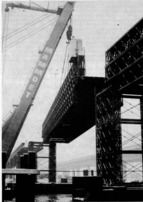
Photo 4. Dismantling the Bailey Bridge
