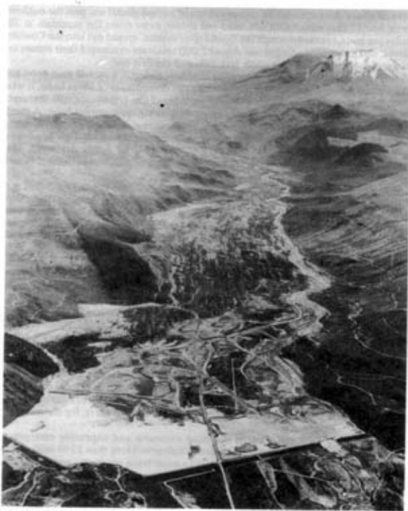
Photo 6. Recent photo of the mud slide in the North Fork of the Toutle River. The debris retaining structure is in the foreground. The river is presently flooding the North half while the South half is being excavated. The darker texture on the end of the mud slide is due to successful aerial seeding designed to stabilize the material. In the background the crater (some 14 miles away) is still slightly active
