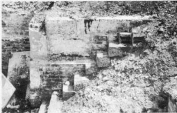
Figure 5. Steps at Newhaven showing Brick Aggregate for Concrete in Tension
