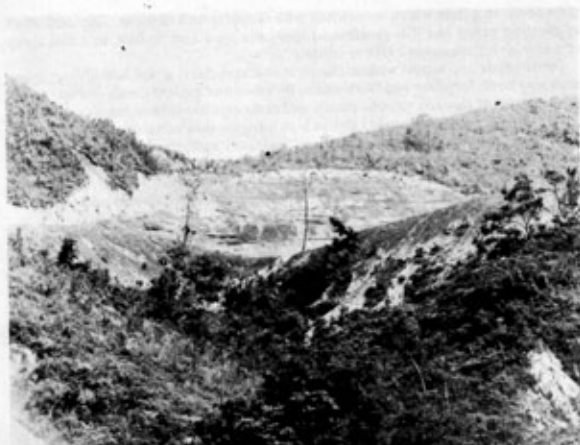
Photo 3. The borrow area cut slope two weeks after seeding. Note the temporary boards erected to prevent wash-down of fine material
