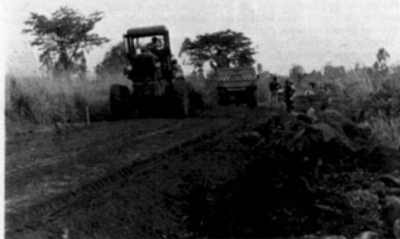
Photo 9. Grading imported fill on the road
