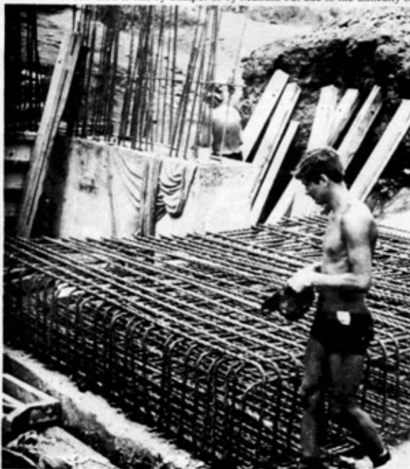
Photo 4. Cage reinforcement for the raised wing wall foundation
