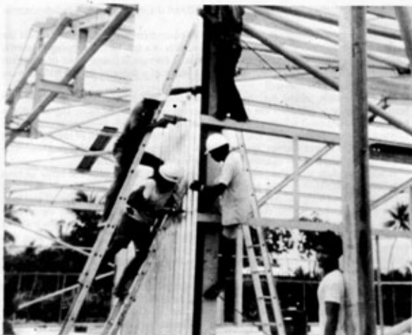
Photo 4. Fixing Cladding
