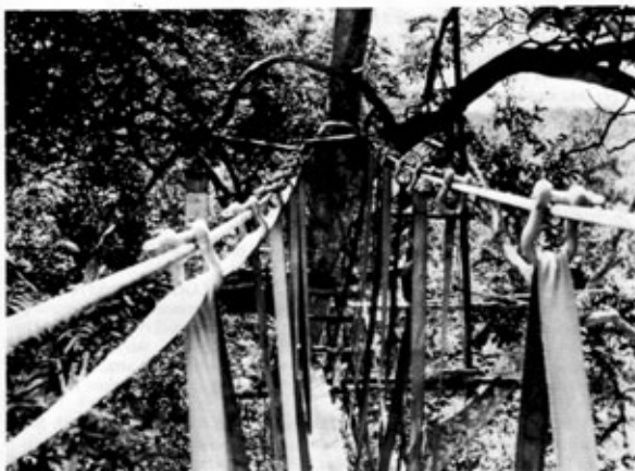
Photo 1. The end of the walkway showing the platform and the diagonally arranged safety strapping. The box suspended to the left of the walkway is an insect trap
