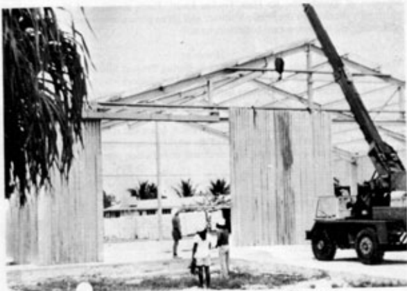
Photo 5. Hanging Modified Doors using 6 Ton Iron Fairy Crane
