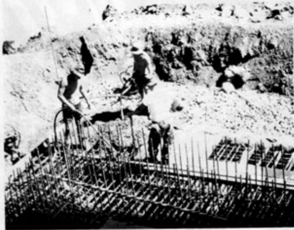
Photo 3. Poker vibrators being used on the abutment foundation on the west bank. Note use of gabion boxes as formwork
