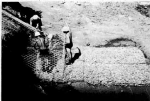
Photo 1. Hand filling of gabion boxes
