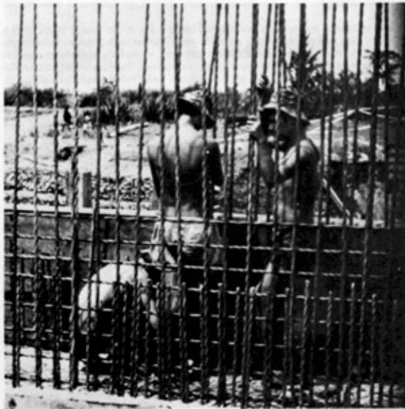
Photo 6. Tying-in horizontal reinforcement on west abutment
