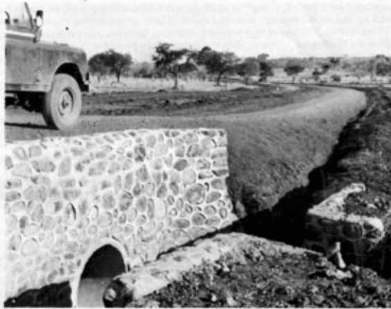
Photo 10. Typical culvert, 900mm pipe and random stone walls
