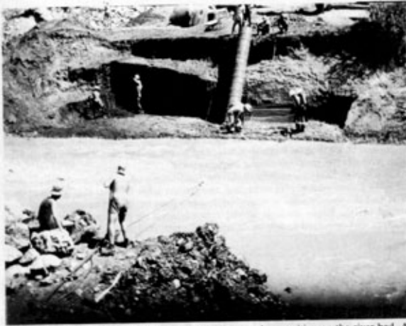
Photo 2. Using a Tirfor jack to winch gabion mattresses into position on the river bed. All excavation was by hand
