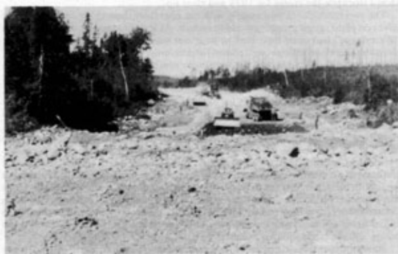
Photo 2. Work in progress on the roads. In the near distance is a minor dolerite outcrop which was levelled by drilling and blasting. The difference in vegetation on either side of the alignment is due to a forest fire five years ago. A logger had cleared the road alignment which acted as a fire-break.
