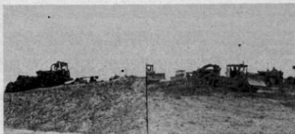
ABOVE LEFT A TEREX DUMPING ON THE TOPSOIL STOCKPILE RIGHT D6C WITH 8 CU YD SCRAPERS STRIPPING TOPSOIL BELOW TOP AN AVRE PUSHLOADING A TEREX MOTORISED SCRAPER CENTRE A D6C PUSHLOADING A TEREX MOTORISED SCRAPER BOTTOM A D6C TOWING AN 8 CU YD SCRAPER BEING PUSH- LOADED BY A D6C TOWING AN 8 CU YD SCRAPER BEING PUSHLOADED BY A VICKERS
