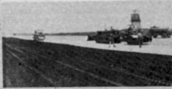
ROLLING THE LOPSTONE RUNWAY EXTENSION WITH A 6/8 TON STOHERT AND PITT VIBRATING ROLLER AND GRADING THE TOPSOIL BAND AREA.
