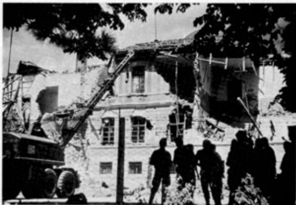
Photo 4. Mobile crane adapted for use as battering ram.
