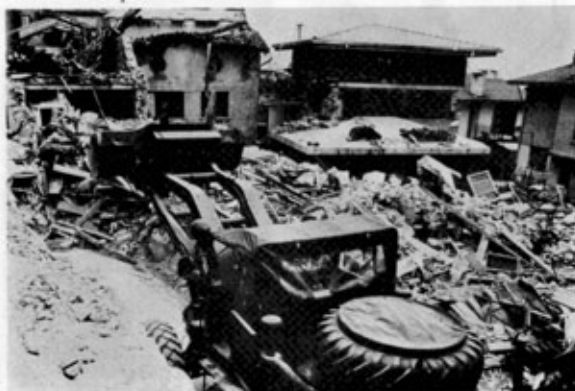
Photo 6. FAG Medium Wheeled Tractor clearing rubble in Gemona.
