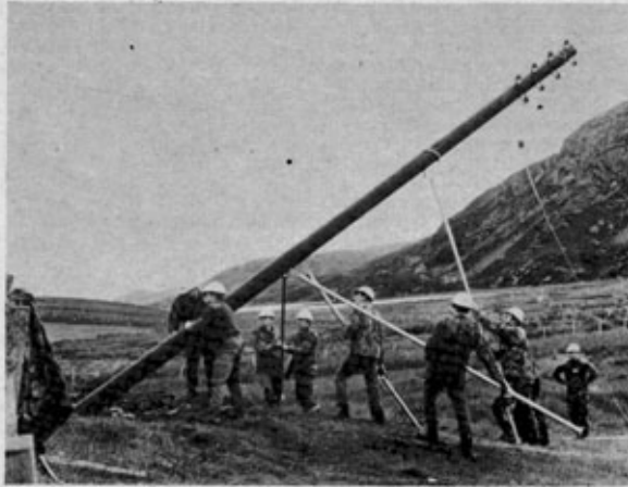
Photo 1. Pole erection using "pikes"
