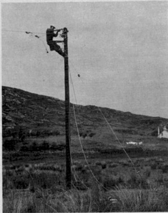
Photo 2. Linesman tensioning conductors on a replacement pole
