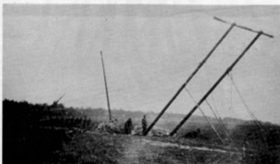
Photo 4. Pylon erection in Lowlands.
