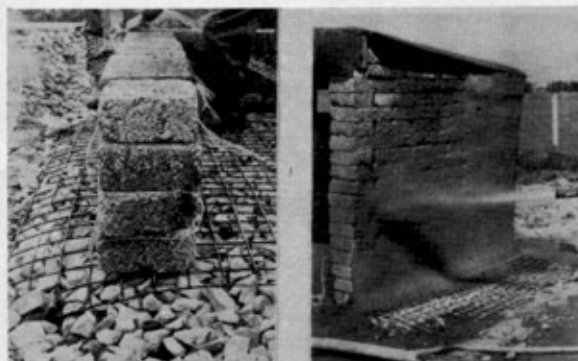
Photo 7 [L and R]. A trial for a sangar/OP. Square Mesh Track was used to give a strongly keyed base. The structure was built in three hours, (designed on site and using materials to hand), and had one open wall and only one embrasure due to imminent withdrawal of the Gunnite equipment and consequent lack of time and materials.
