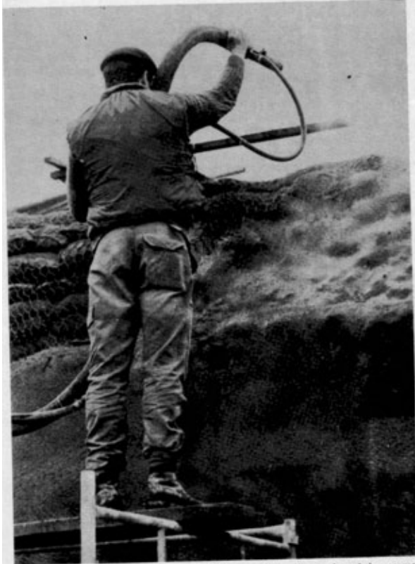
Photo 4. Guniting in progress. Note the chicken-mesh key, the nozzle and the separate pipes for the dry mix and water.
