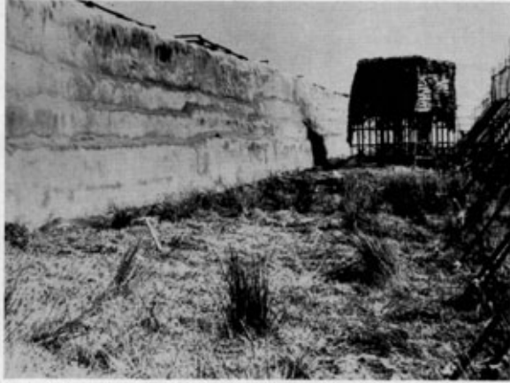
Photo 5. The completed outer face. Just visible over the wall is the mortar protection on the roofs of huts.
