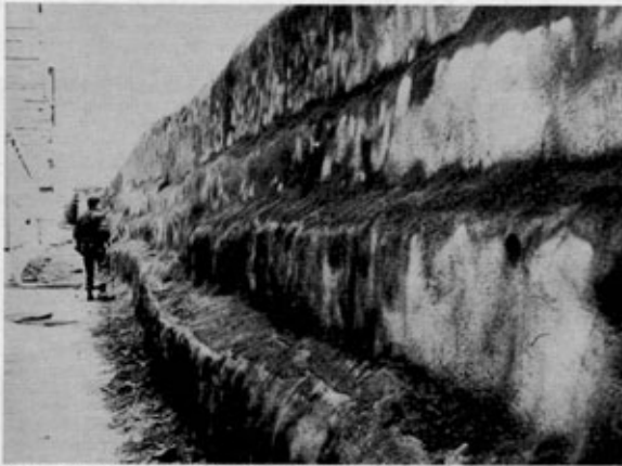
Photo 6. The complete inner face. Note the loose waste which has fallen onto ledges and ground.
