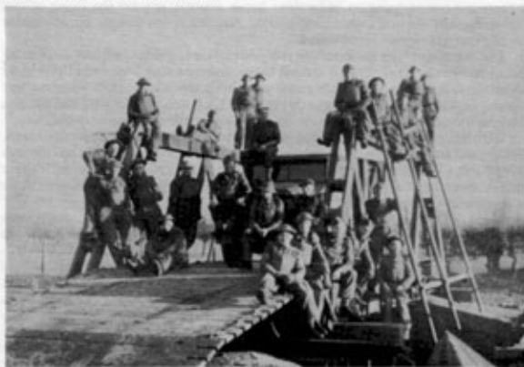
Photo 1. 32ft span truss bridge made up from chesses.
