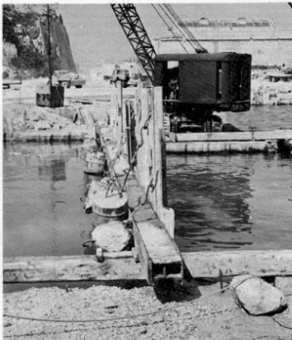
Photo 2. Arrangement of formwork.
