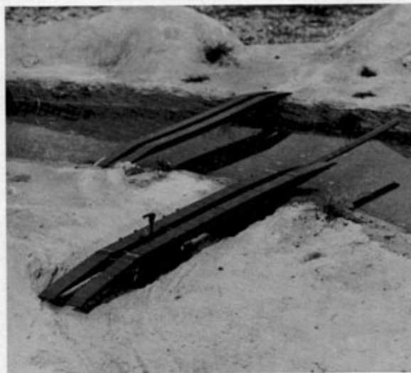
Photo 2. Wheeled Transporters Connecting two long bridge sections for launching.
