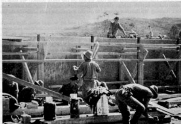
Photo 4. Butt wall under construction.
