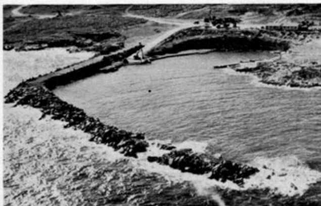
Photo 1. Akrotiri Mole after the severe storms of Winter 1968/69.
