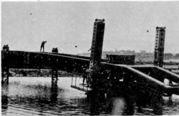
Photo 3. Gundolph Pool—Offshore pier boomed forward.
