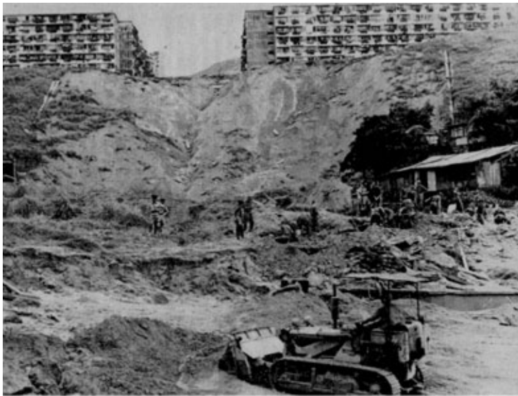
Plate 2. The landslide at Kun Tong. The tufts of grass in the foreground have slid undisturbed from the top of the slope. The earth beneath them engulfing squatter shacks similar to that on the right.
