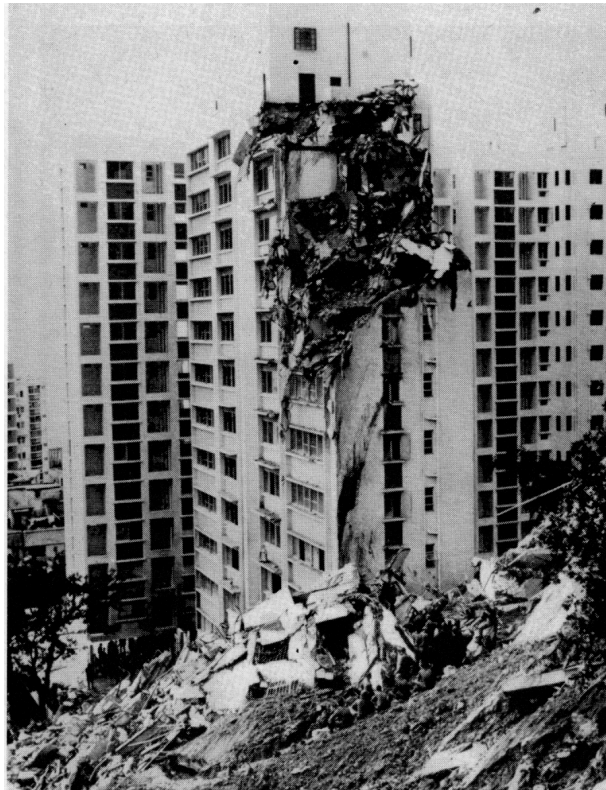
Plate 3. Kotewall Road. In the foreground the remains of a twelve-storey block of flats lie buried in the fall and a working party pauses briefly in digging for victims. Above is a similar building also damaged as the shattered block fell past it.
