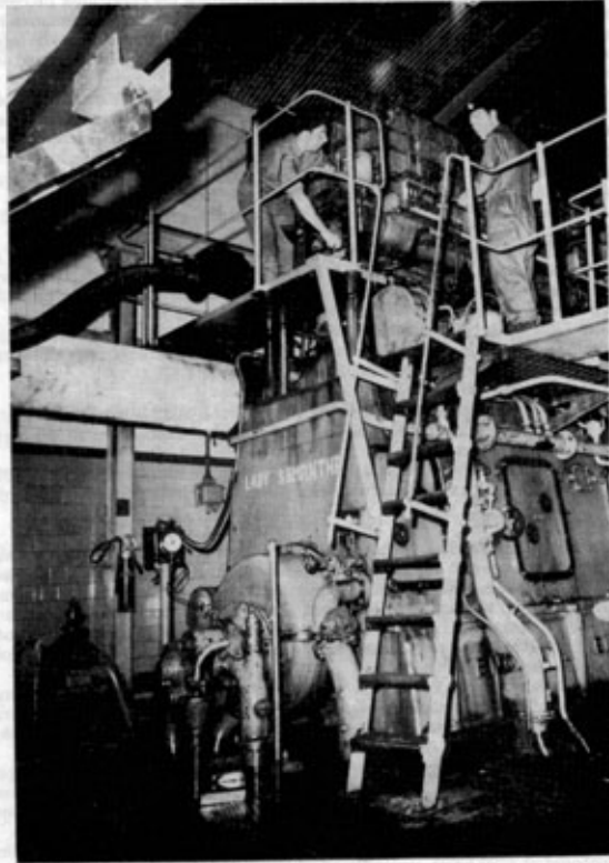
Photo 2. S/Sergeant G J McAllister and Corporal R G Jones fault finding on the diesel engine.
