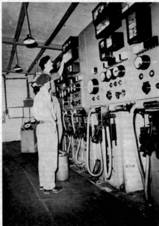
Photo 1: 2nd Lieutenant J M G Hendry and S/Sergeant P E R Shilling (64 CRE) checking the high voltage protection.
