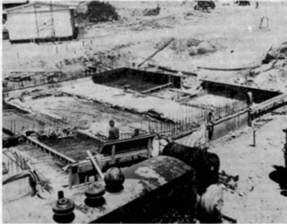
Photo 4. General view of the deep end of the pool. The centre bay in the picture has just finished its last stage of curing, ie ponding, and the sandbag dam and hessian are being removed. The central bay on the left had been poured the night before and the stand off hessian frames are in position.
