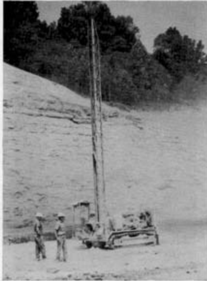
Plate 8. Self-propelled crawler drilling rig seen here drilling 43-in diameter primary holes. Pre-Split surface in background.
