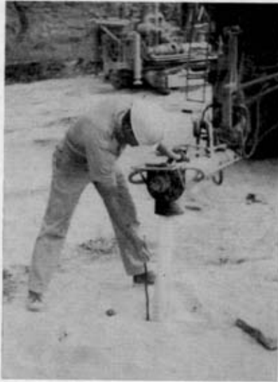
Plate 1. Mixture of Ammonium Nitrate and Diesel being poured into a dry primary hole. Stick being used to measure depth of fill.
