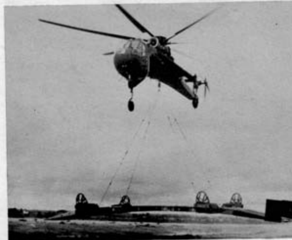
Plate 3. CH 54A Carrying CI 16 (APB) Raft complete.
