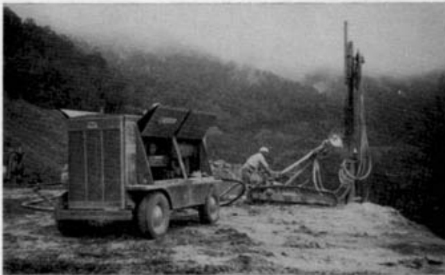
Plate 9. Small bore crawler drilling rig with accompanying air compressor to provide power.
