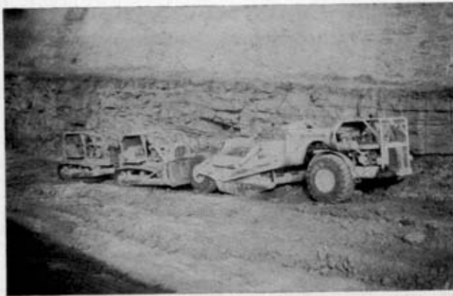
Plate 7. Scraper being used after blasting using Pre-Splitting. Note how it can work close to the rock face.
