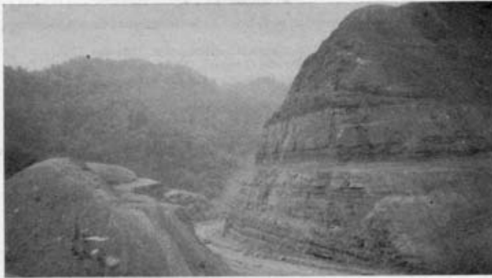
Plates 10 and 11. Examples of Pre-Split cuttings during the construction of Highway 15 at Carr Fork, Eastern Kentucky, USA.
