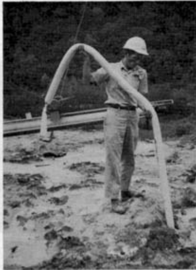
Plate 2. Ammonium Nitrate in protective polythene tube being loaded into wet primary hole.
