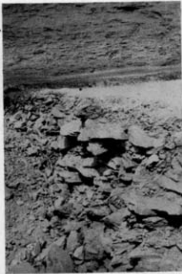
Plate 6. Foreground: Shows face left after primary blast with no control blasting techniques used. Background: Top of photo shows face left by Pre-Splitting in the same rock.
