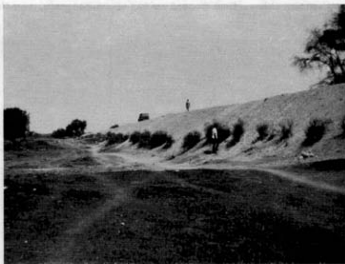
Plates 2 and 3. Part of the Garissa Causeway showing flooding on the upstream side and 18 ft of fill downstream.
