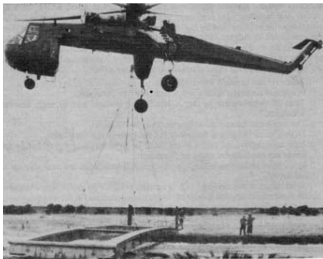
Plate 6. CH 54A Emplacing 80 ft SS MGB undecked.
