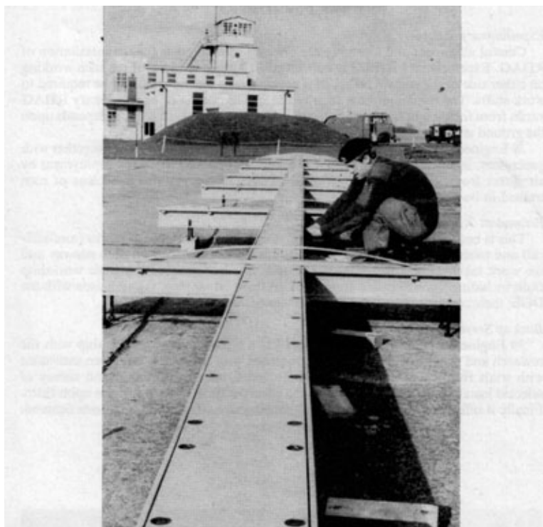
Plate 12. The retractable hookcable support system undergoing assembly trials at WATER-BEACH in February 1972.
