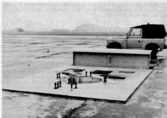
Plate 2. Base foundations and switch board for a permanent EAU at RAF MANSTON.
