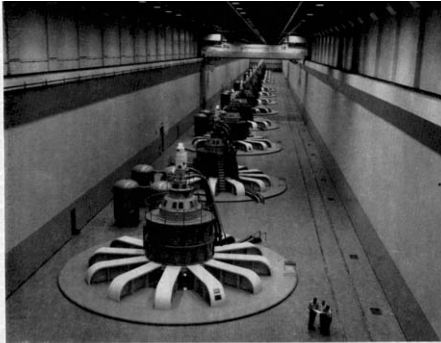
Plate 10. The Dalles, Oregon. Interior photograph of the powerhouse at the Dalles Dam. When installation of eight new units is completed the powerhouse will extend from its present 1,462 ft length to 2,150 ft. The generators shown have nameplate ratings of 78,000 kilowatts each. The room housing the generators is 75 ft wide and 73 ft high.
