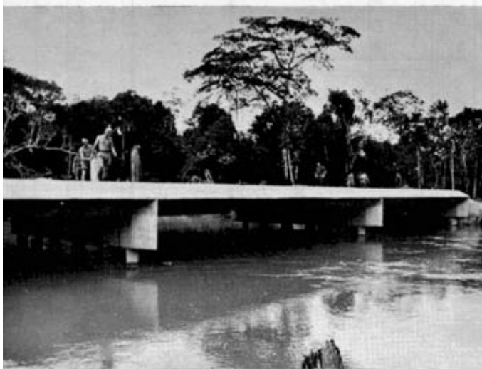
Plate 10. Bridge 2. Expansion joints are sealed on the completed bridge
