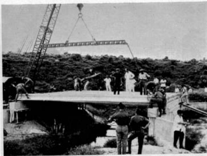
Plate 6. Bridge 1. The last prestressed concrete beam is placed during a visit by the Deputy Prime Minister of Malaysia
