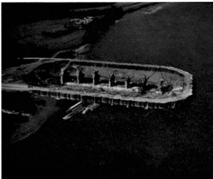
Plate 3. Cannelton River, Ohio, Kentucky Bank. Dam construction inside cofferdam.
