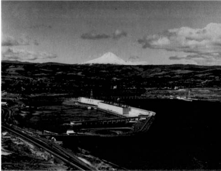
Plate 8. The Dalles Oregon. The Dalles Dam on the Columbia River with Mount Hood (11,235 ft) in the background. The navigation lock with a lift of 87.5 ft is on the right, the powerhouse parallels the river at the center
