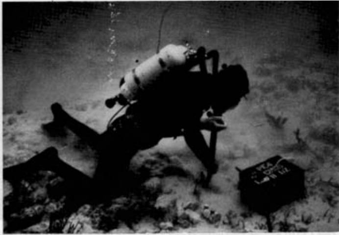
Plate 3. Digging in charges from holes loosened by CD11 action; 40 lb PE4 is about to be buried
