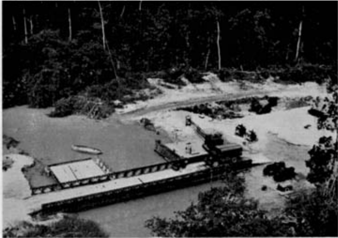
Plate 7, Bridge 2. A temporary access bridge and piling platforms can be seen. The wet piers have been piled and capsills are being constructed
