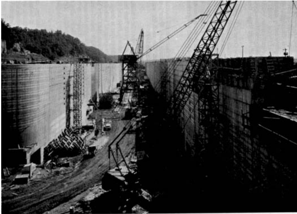
Plate 2. Cannelton, Indiana. Construction of lock
