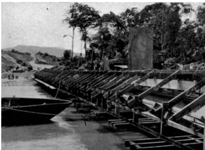
Plate 9. Bridge 2. Shuttering being fixed for the pointed cutwater
