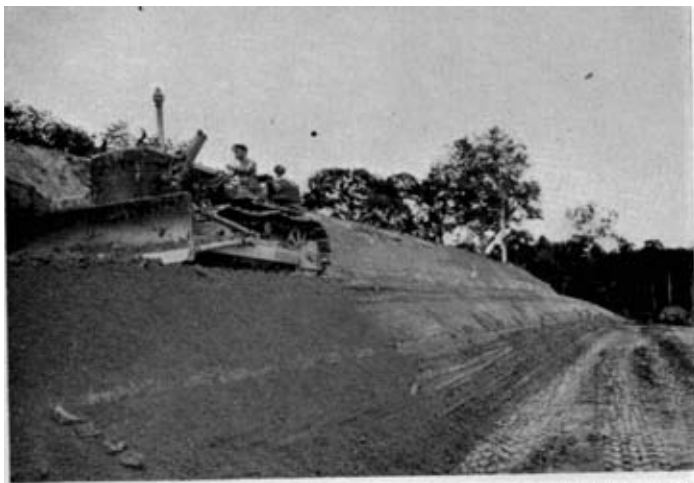
Plate 5. Earthworks in progress on the road. Banks of cuttings over ten feet in height were benched
