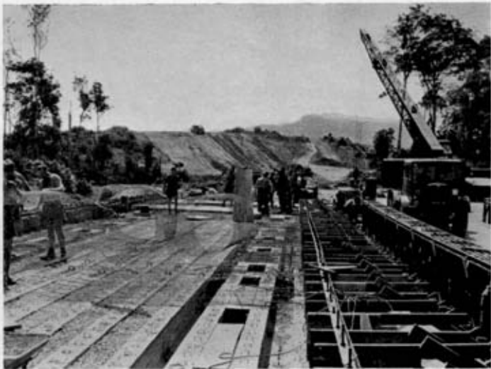
Plate 8, Bridge 2. Reinforcement mesh being laid for the deck slab
