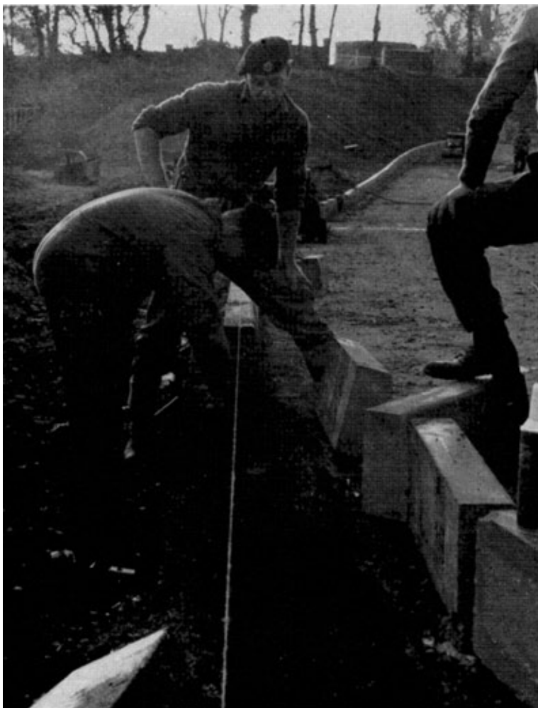
Photo 4. Kerb laying in Church Crossing area.
