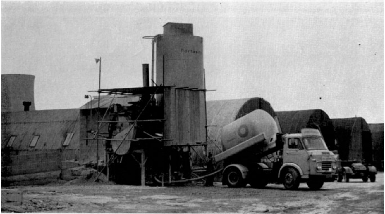
Photo 5. The mixer arrangement and steam plant. Note: The steam plant is so situated that it can be used for de-icing the aggregate in winter.
