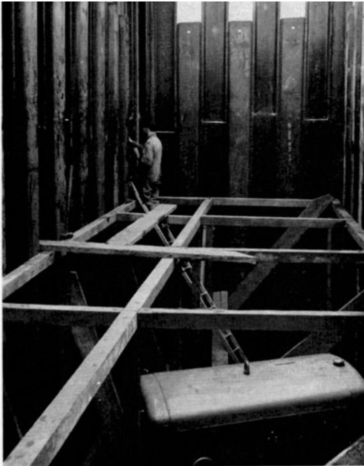
Photo 6. Welder at work inside Cofferdam.
