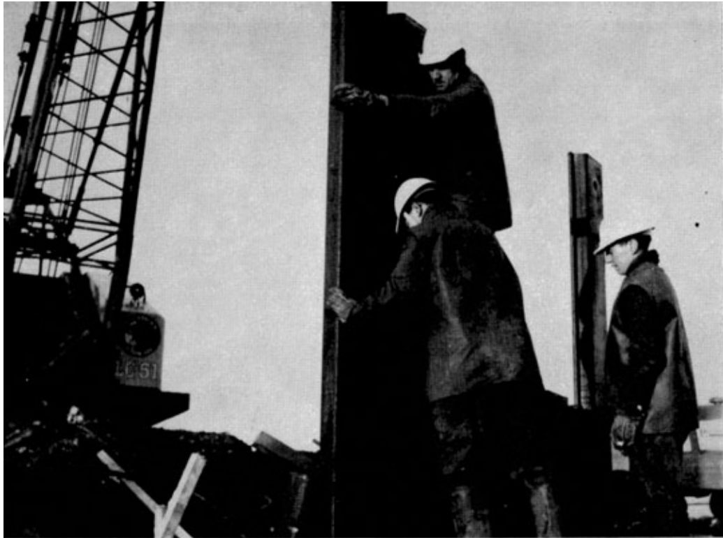
Photo 3. Piling the end dam. A timber piling frame was used for the first eight piles at each end.
