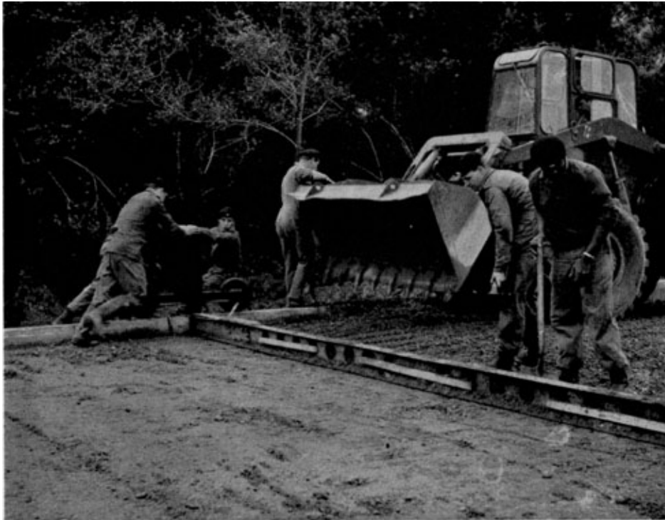
Photo 3. Spreading the dry lean base with Michigan, and final levelling with the Travelling Screed Board on the kerbs.
