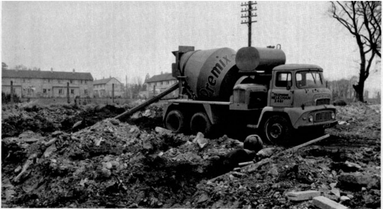
Photo 7. Truck mixer M5P by Stothert and Pitt Limited. Delivers 5 cu yds of dense concrete, and can be petrol or diesel engined. The mixer can be put on a wide range of approved chassis.
