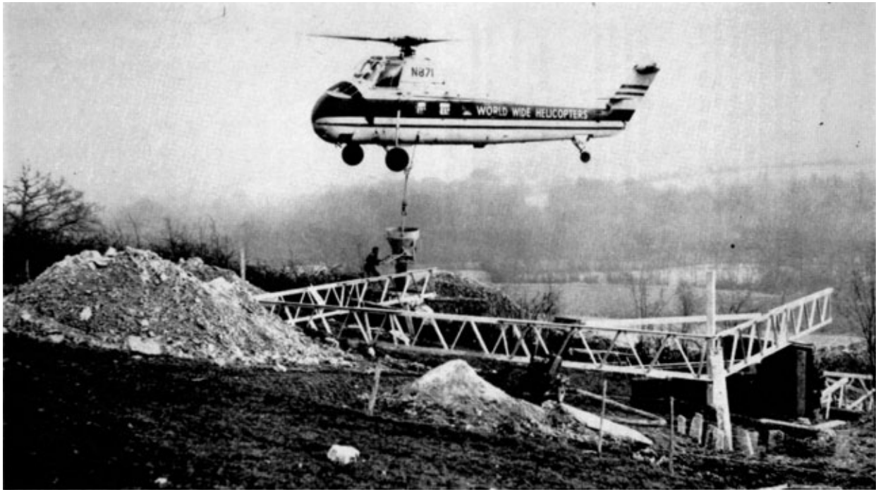
Photo 8. In 1964 concrete foundations for electricity pylons were constructed by delivering ready-mixed concrete by road to selected points, and then air-lifting it in lightweight Audax 12 cu ft "Dual Flow" skips to the erection area.
