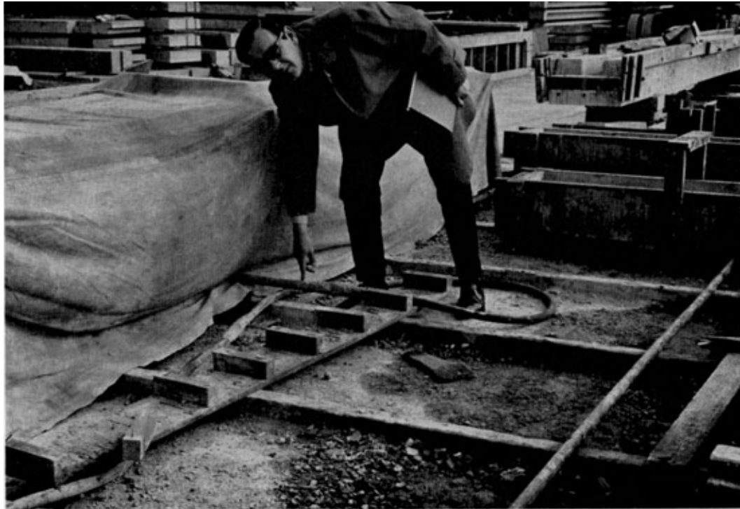
Photo 3. A group of moulds under a canvas sheet. Here one can see the steel pipe used for steam distribution, and the rubber hose connecting from the main to a second steel pipe under the mould. The holes in the steel pipe are \frac{1}{4} in diameter and at 18 in spacing.
