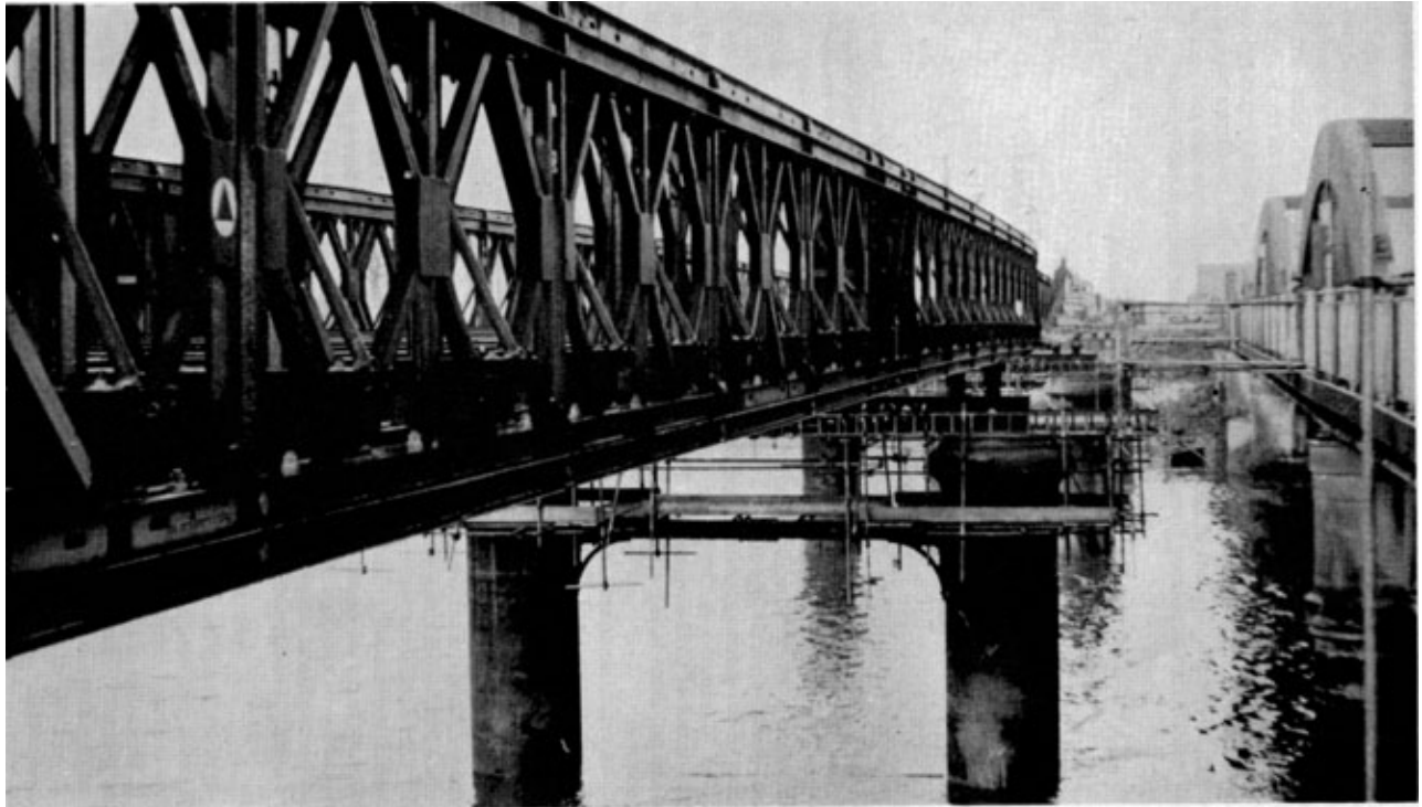
Photo 4. The bridge during launching. The scaffolding off the Cut Bridge enable concrete and roller assemblies to be carried on to the piers.
