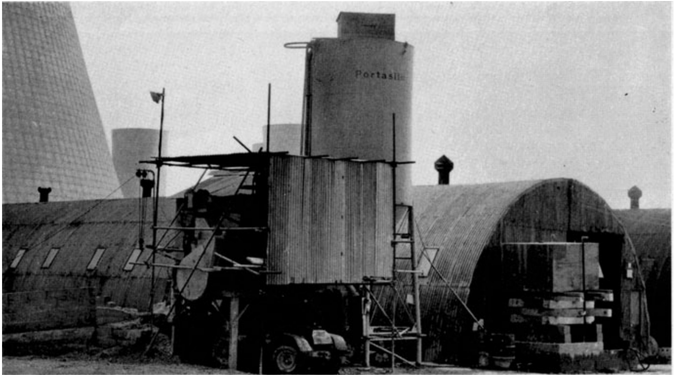
Photo 4. A general view of the site factory showing the converted Romney huts, the type of unit cast, the mixer arrangement, and behind it the steam-raising plant.
