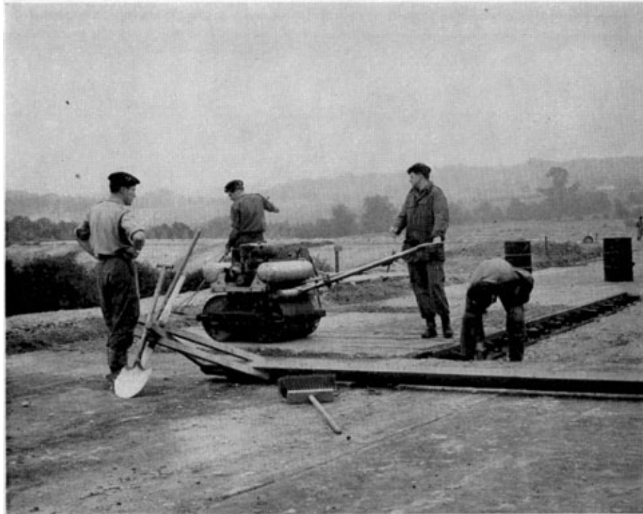
Photo 2. Final compaction of the cement bound granular sub-base with Bomag vibrating roller.
