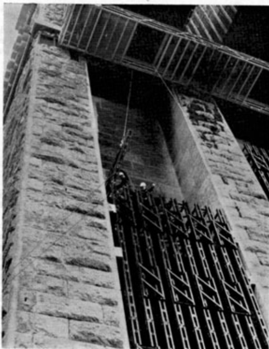
Photo 5. The first panel of the fifth lift being lowered into position—Caernarvon Pier
