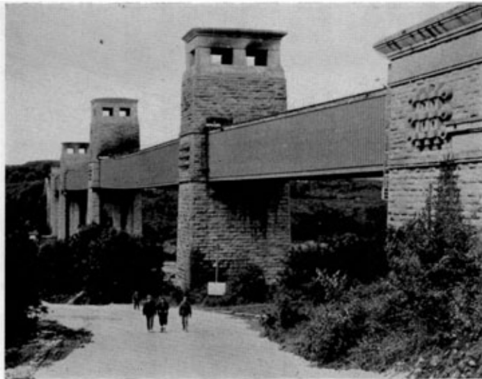
Photo 1. Britannia Tubular Bridge from Caernarvon Abutment, showing the sag in the tubes
