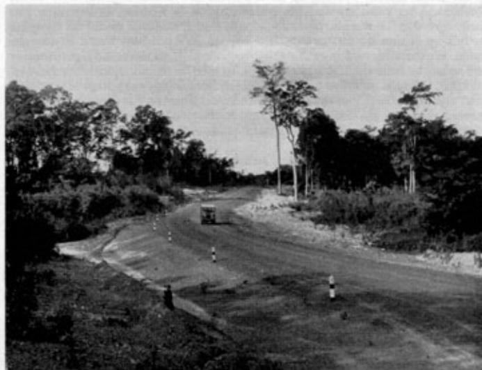
Fig 8. The completed road at the twenty-second kilometre, known by the Force as "the escarpment". It was along this stretch that 11 Independent Field Squadron did considerable blasting of rock and trees, using Prilled Ammonium Nitrate. (See "Use of Prilled Ammonium Nitrate as an Explosive", by 2nd Lieutenant I. J. K. McLean, RE Journal , September 1968.)
