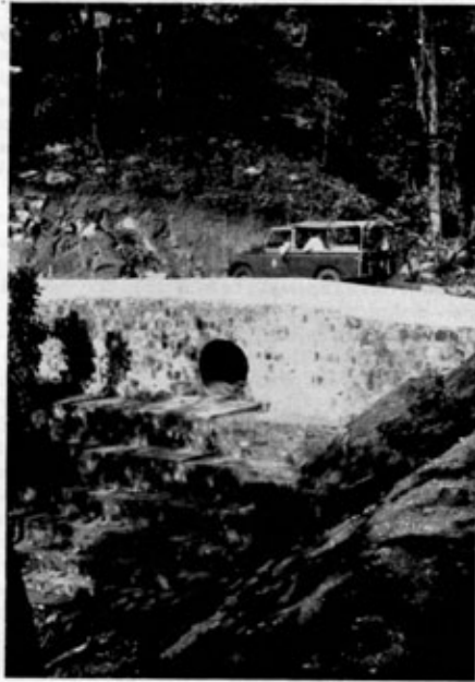
Large culvert with anti-erosion steps.
