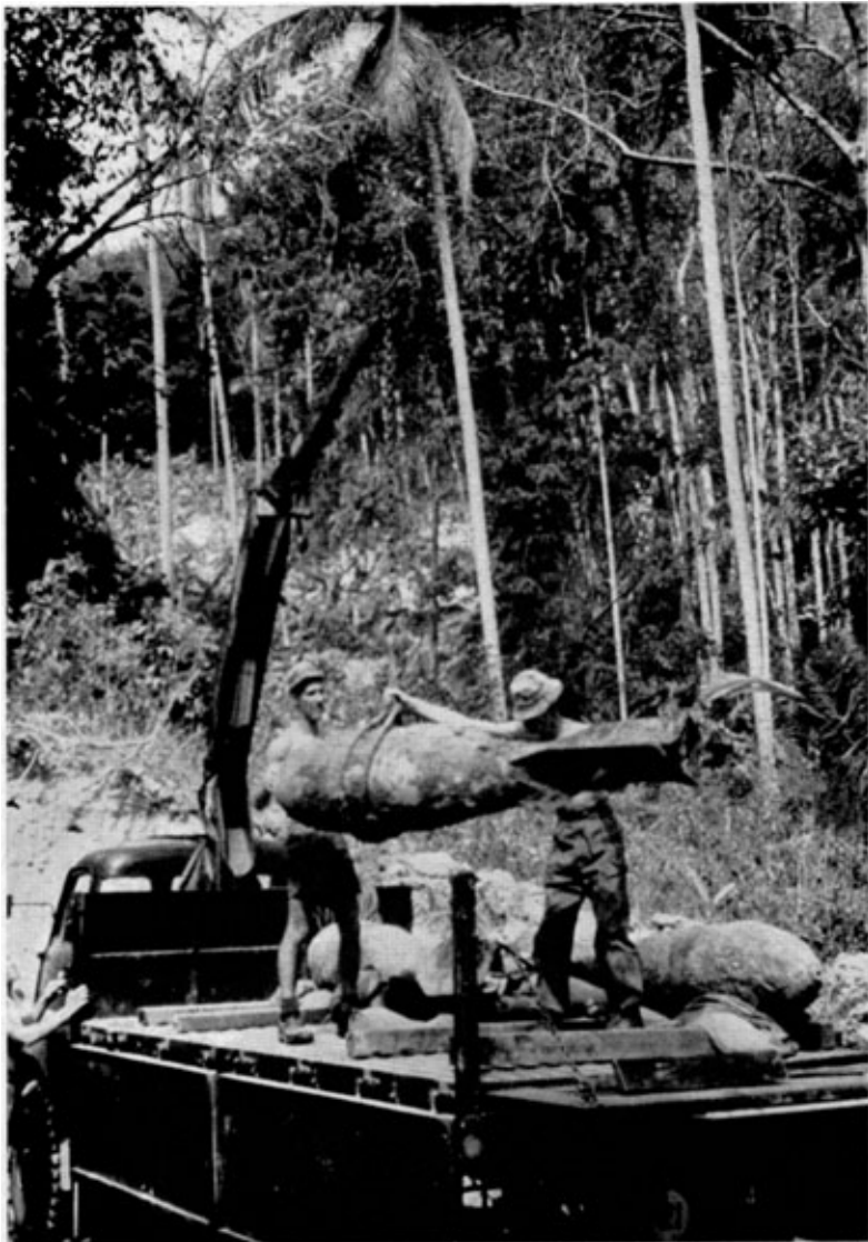
Photo 4. Loading a 500-kg bomb on to a truck with the Hiab crane, site 2, Sungei Dua Dua. Two bombs have been loaded already and are chocked with sandbags.
