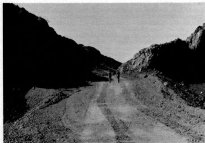
Fig 8. Wadi Matlah—an example of the amount of rock blasting necessary to keep the alignment out of the Wadi Bed—(named “Fitz Polly” by 48 Field Squadron as a token of respect for their OC).
