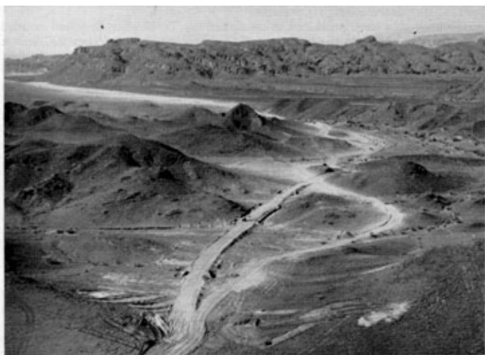
Fig 5. The northern sector—three miles south of Al Milah—culverts completed and formation under construction.
