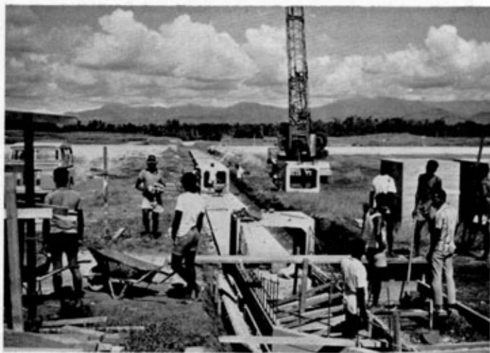
Photo 4. Constructing a cross culvert under the runway and flight strip with precast sections.
