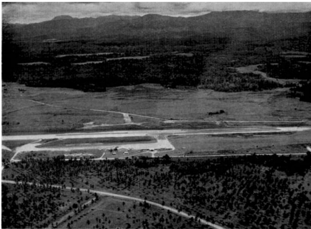
Photo 1. Henderson Field, Guadalcanal. View from the north, September 1968, showing the eastern half of the runway rebuilt, but not yet with its bitumen surface.
