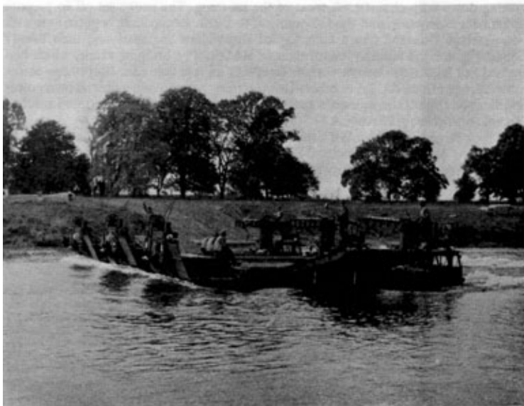
Photo 2. A three rig M2 ferry, capable of carrying Class 60 loads.
