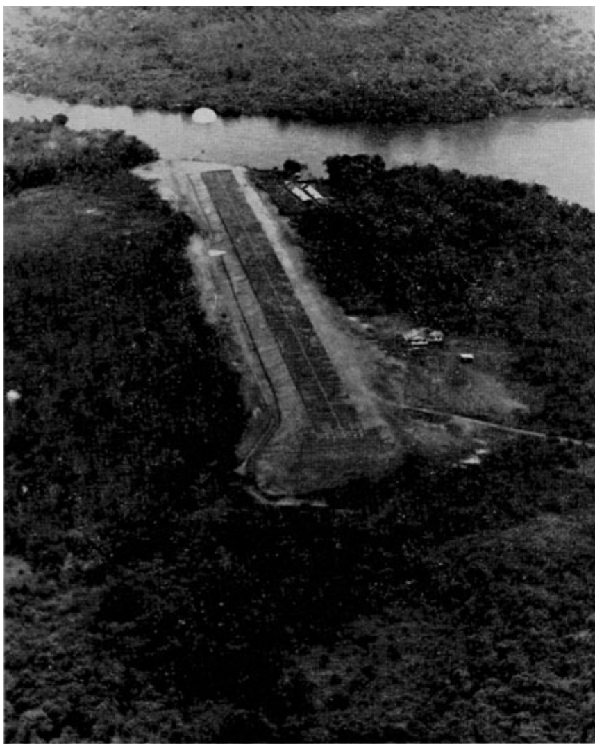
Photo 6. Long Akah airstrip. Originally a mission strip, rebuilt by 69 Gurkha Indep Fd Sqn after an accident to a Twin Pioneer. Plant for the task was air dropped, the PSP was brought in by long boat.
