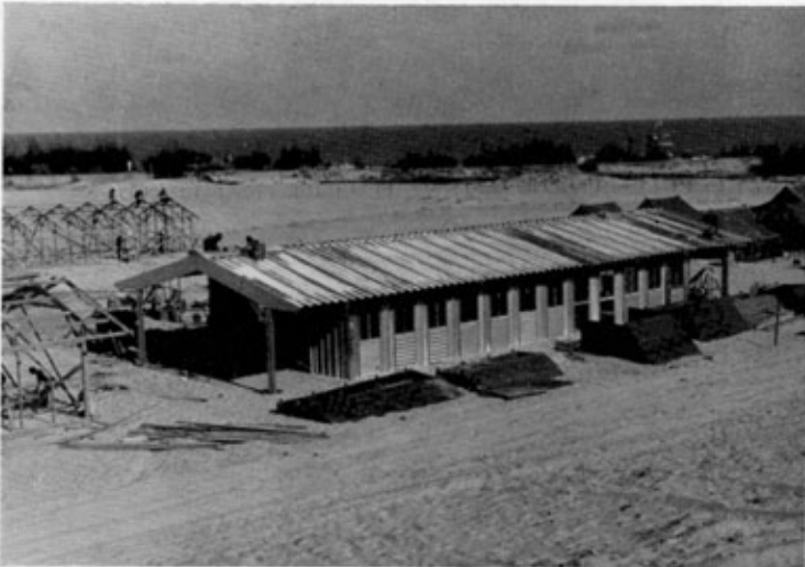
Fig. 7. Galvanized iron prefabricated office building under construction by Sappers. Normal building time forty man days (including concrete).
