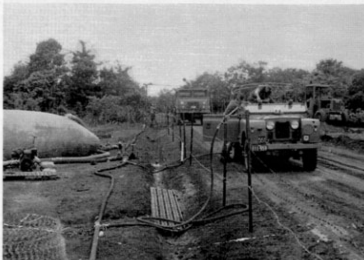
Fig. 3. Task Force water point at early development stage. The petroleum handling piping and pumps permitted fast issuing to vehicles.
