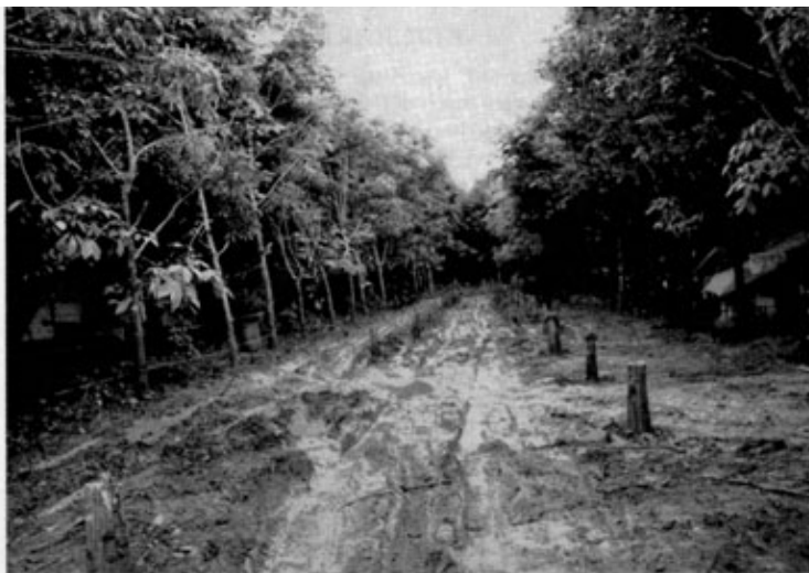
Fig. 8. Road alignment prior to arrival of sappers. Trees were cut by unit labour to assist with drying out.
