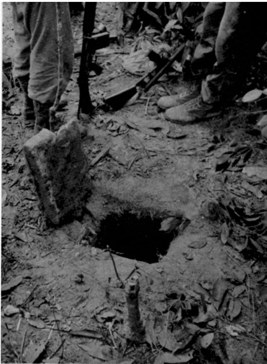
Fig. 1. Entrance to VC tunnel system. The trap-door lid was cast in concrete.
