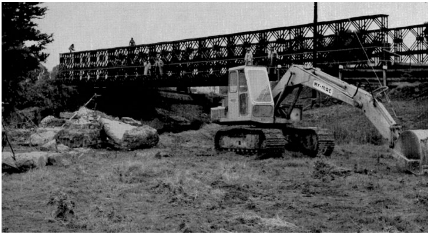
Photo 1. 120 ft Triple Double EWBB Class 70 built by 20 Field Squadron RE at Fenny Bridges.
