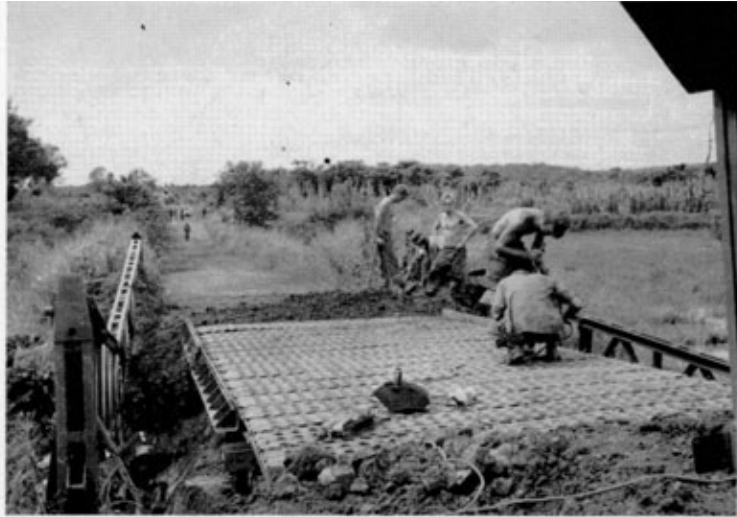
Fig. 4. Expedient replacement of Bailey Bridge blown by VC. Timber bearers, and partly damaged transoms were used with PSP decking.
