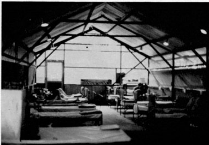
Fig. 2. Task Force area—Field ambulance ward. Galvanized iron and timber structure with insect screening.
