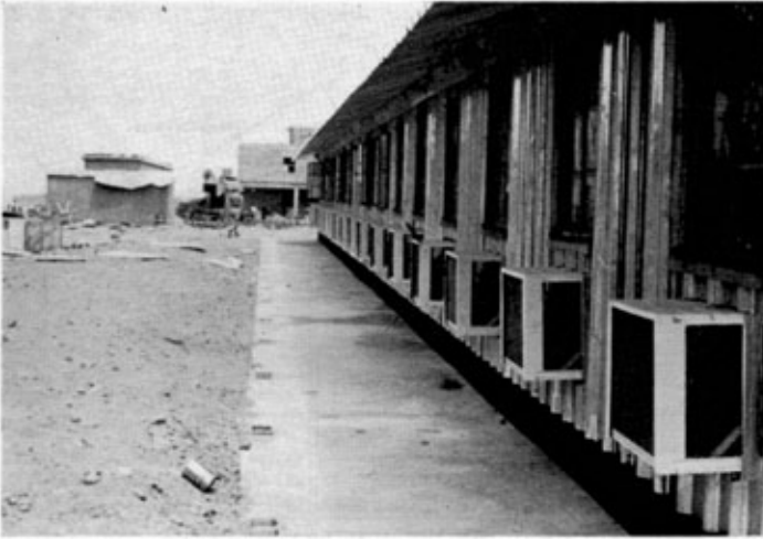
Photo. 5. The Cantonment, Mareth Lines. A battery of 1 ton air-conditioning units installed in a 128-ft Twynham hut.
