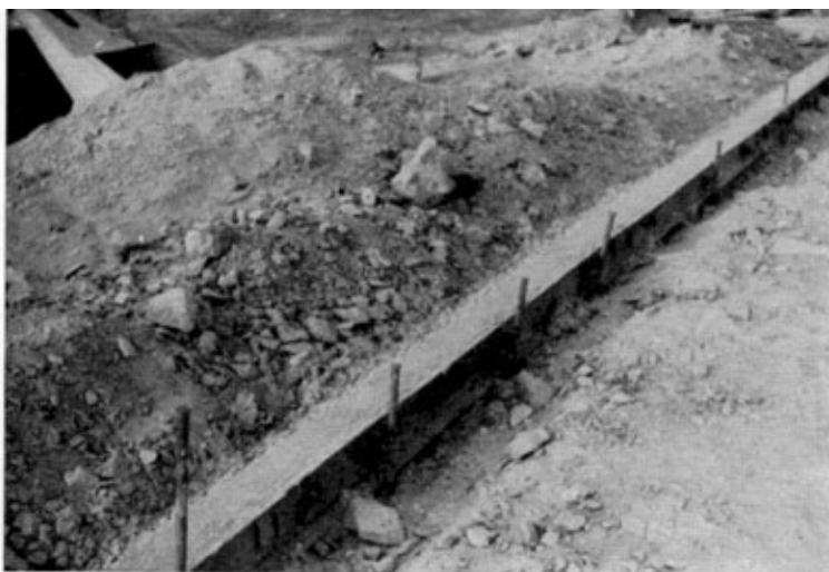
Photo. 16. Jebel road. Method of concreting flush kerbs with shuttering on one side only, set 2\frac{1}{2} in above natural soil level. This method was used on the construction of all roads.
