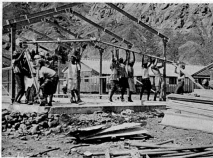
Photo. 13. Twynham hut frame erection at Anzio.
