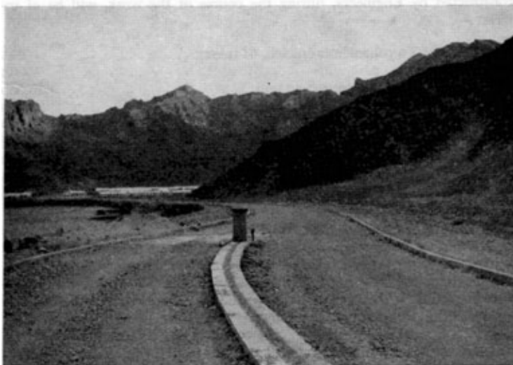
Photo. 15. Same view, after concreting the centre up stand kerb on a dual carriage-way curve.
