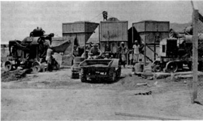
Photo. 3. Normandy Camp. The batch mixing plant in operation.
