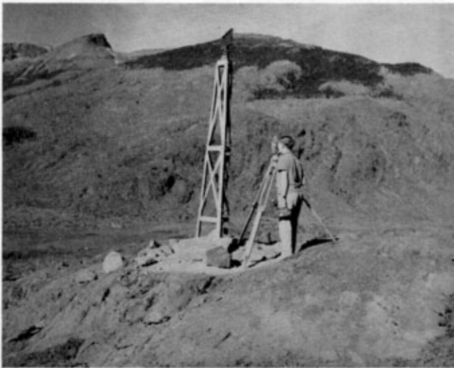
Photo 4. The author siting BP VII-2J on the straight line between BP VII-2H, in the picture, and BP VII-2K on the far side of the Salto/Engano valley. A "handie-talkie" radio is being used to direct Staff Sergeant Browning to the correct location.
