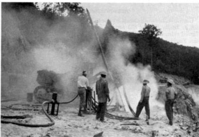
Photo. 2. Drilling a 100 ft borehole. The drill uses 600 cu ft air/min. It has a separate air motor for rotation and special "retrac" arrangements.
