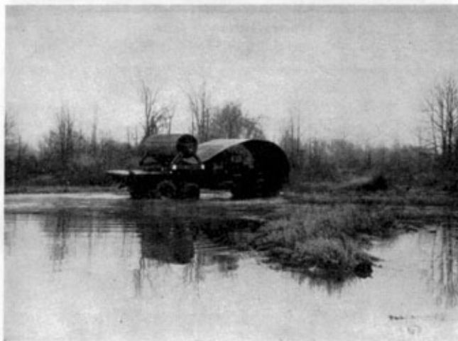
Photo 5. Trackway being launched from American truck bridging 5 ton.
