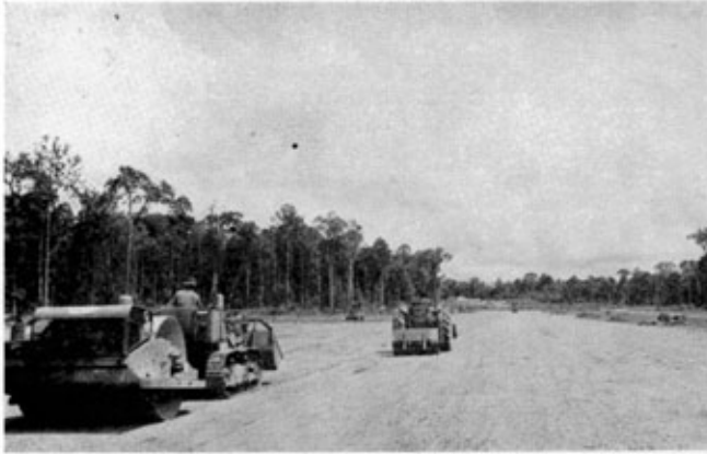
Photo 6. VIBRATING ROLLERS. Two airportable vibrating rollers compacting a new airstrip on Tioman Island in the China Sea. In the foreground is a 72 in, 3½ ton roller towed by a BTD 6 Traxcavator. In the background is a 54 in, 35 cwt roller towed by a Fordson Super Major.
