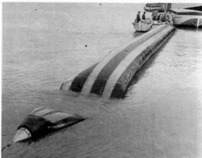
Photo 4. Towed flexible barge—280 tons nominal capacity.
