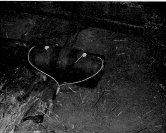
Photo 12. Diamond charge in place (sheet explosive used).
