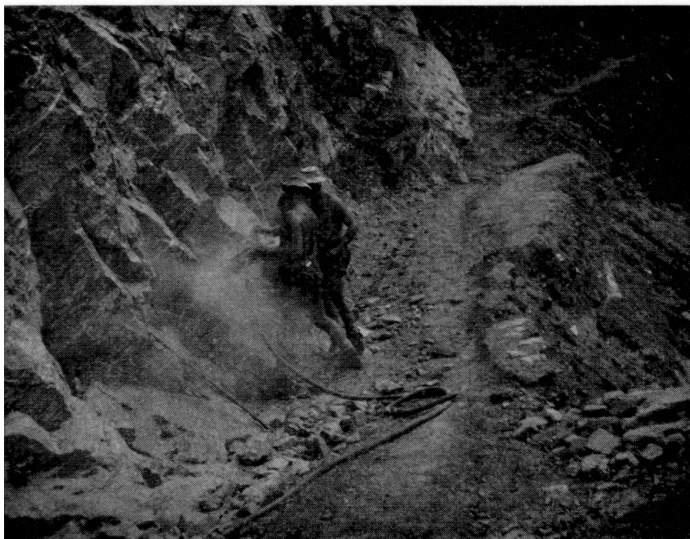
Photo 10. "Drilling and blasting all the way". Sappers of No 3 Troop on the Chesoi-Tot track.
