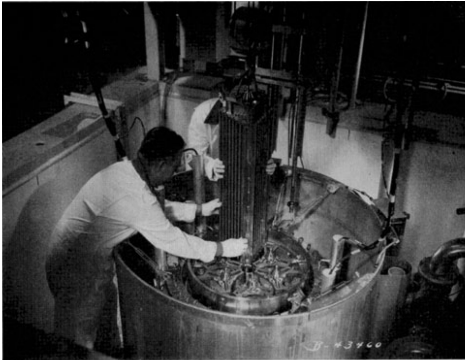
Photo 2. PM-1's CORE IS ASSEMBLED. The fuel load weighs 1,500 lb and continuous full power operation is possible for two years. Two million gallons of fuel oil would have to be burned to release the electrical energy obtainable from a single
