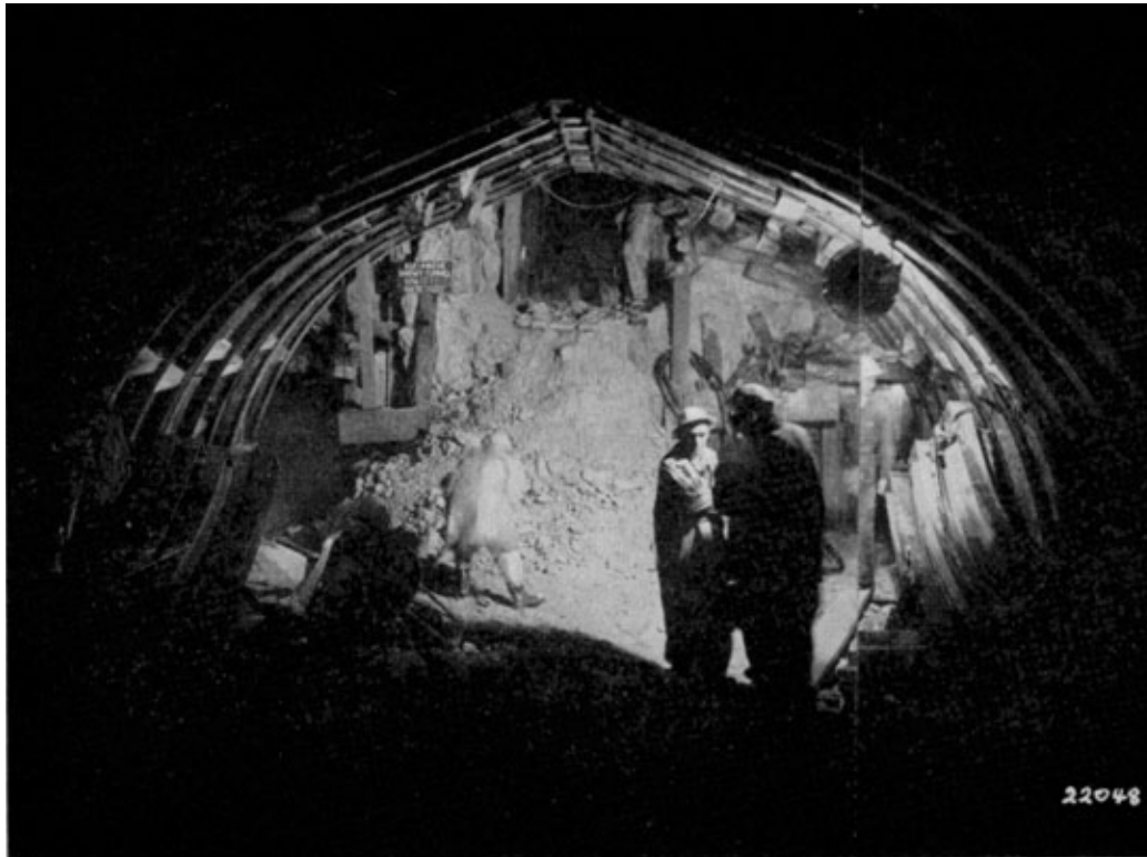
Photo 6. Face at Sta 127 + 17, showing the wallplate and crown drifts
