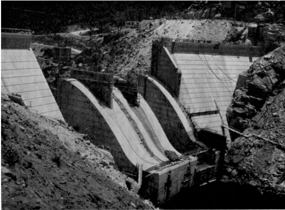
Photo 1. Island Bend Dam, showing the central spillway
