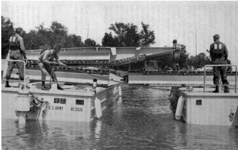
Photo 4. An end bay about to link to an interior bay. (Note the end bay's slightly lower position in the water; and the deckhand preparing to make use of the powered capstan at his feet to achieve the final alignment)
