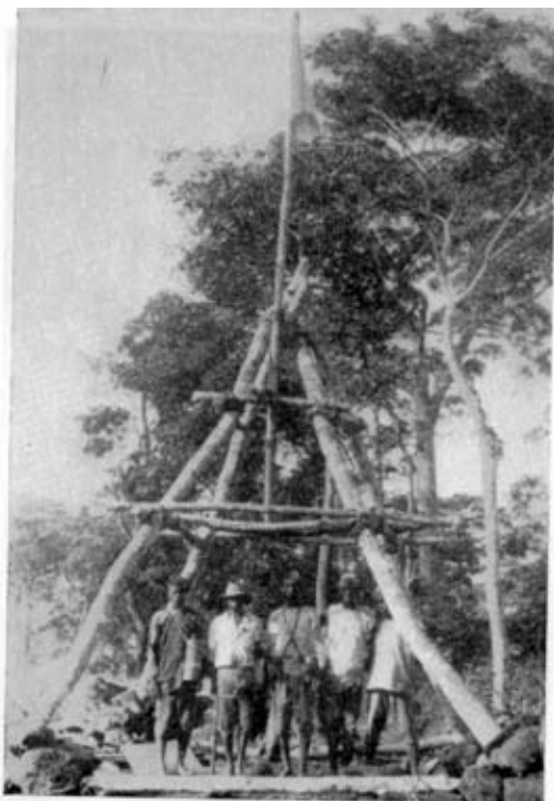
Photo 1. Building a Beacon, or "cockshy" at a MAIN Station.
