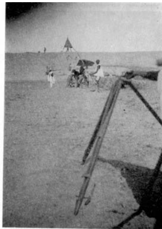
Photo 2. Base Measurement with Invar Tape near Kano.
