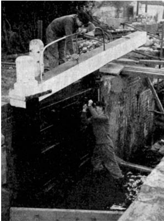
Photo 1. Final fitting of top gate, Lock 31.
