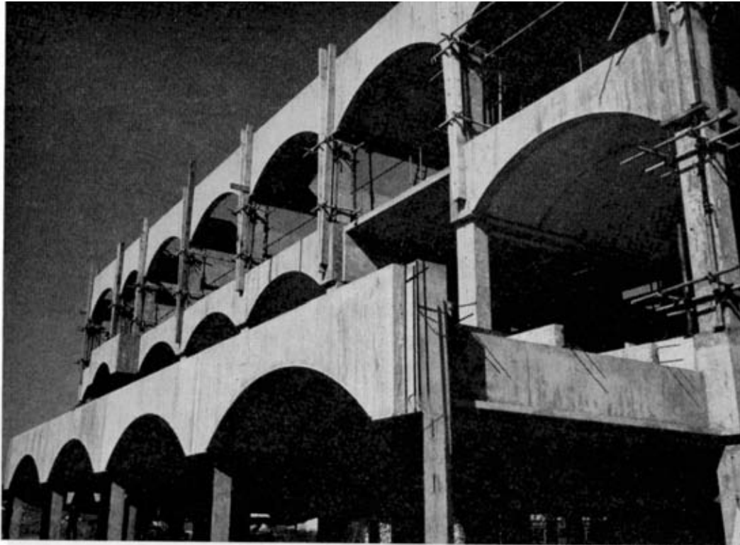
Photo 2. Showing the erection of Main Frame and Vault Units in College House
