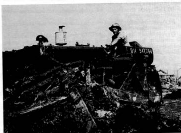
Photo 4. Operating a D4 in Belize. Dozers were used to push the rubble on to the roads where it was picked up by traxcavators and put into tippers.
