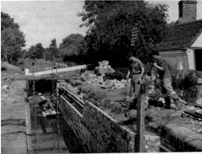
Photo 3. New lock walls back-filled with concrete.
