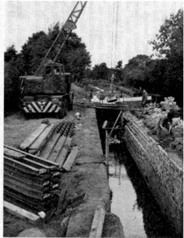
Photo 2. Removal of old coping stones.
